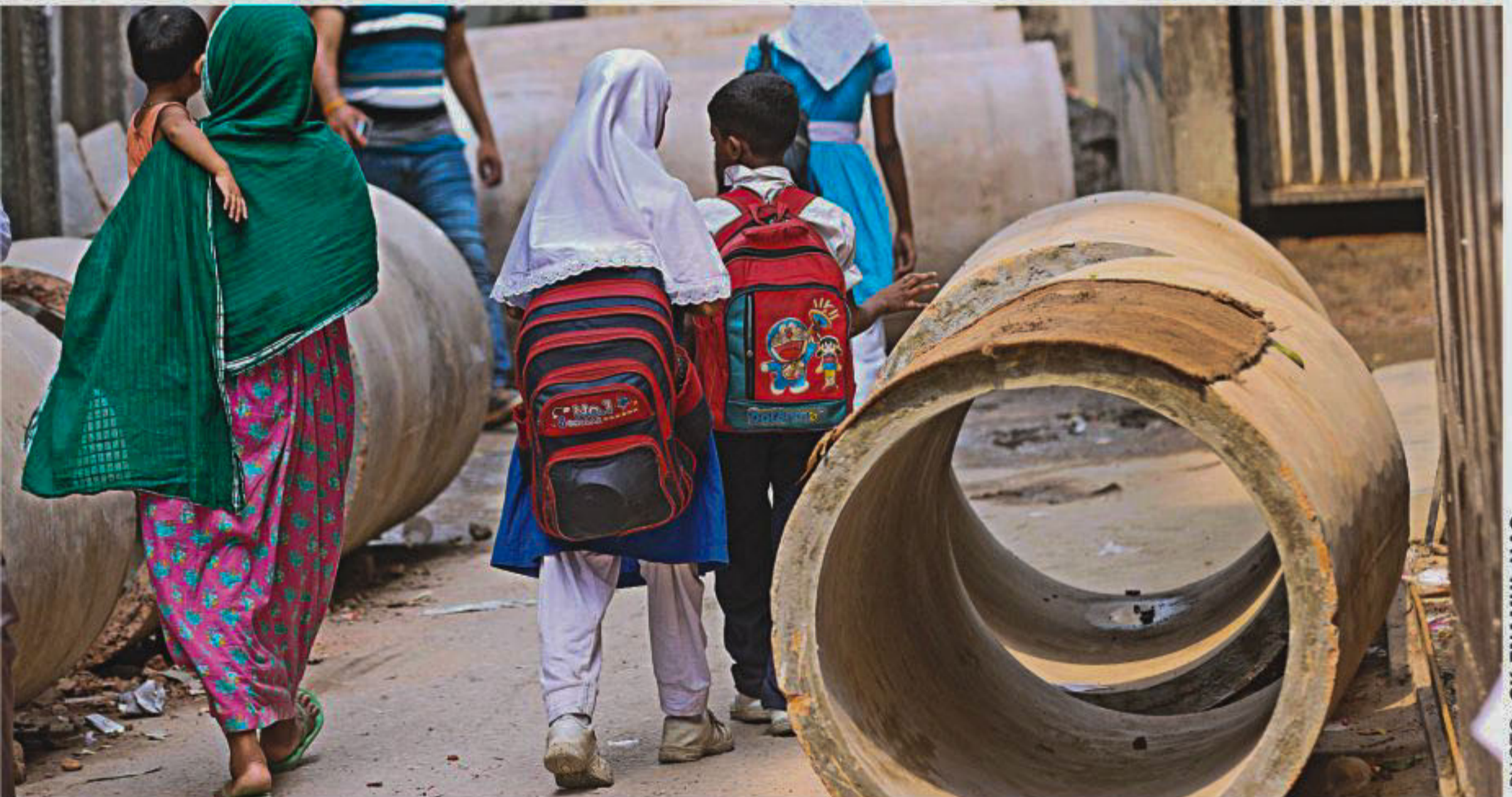
Pedestrians meandering through sewer pipes left haphazardly on the street connecting Madinabagh Wasa Road and Ahambadbagh Road in the capital's North Mugdapara on Thursday, for installing those underground, courtesy of the city corporation south. The situation was still the same yesterday for more than a week.
