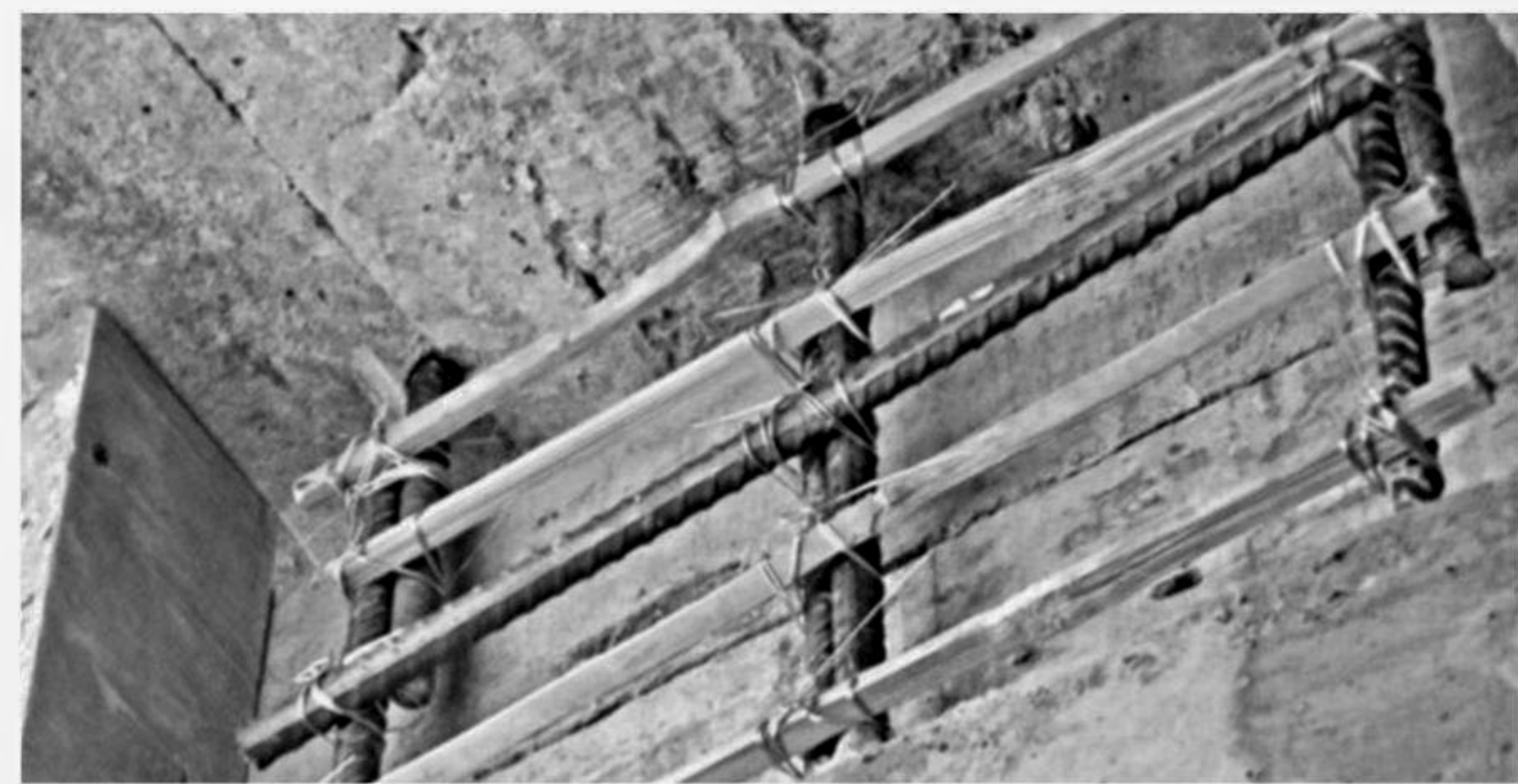
Bamboo, not iron rods...
