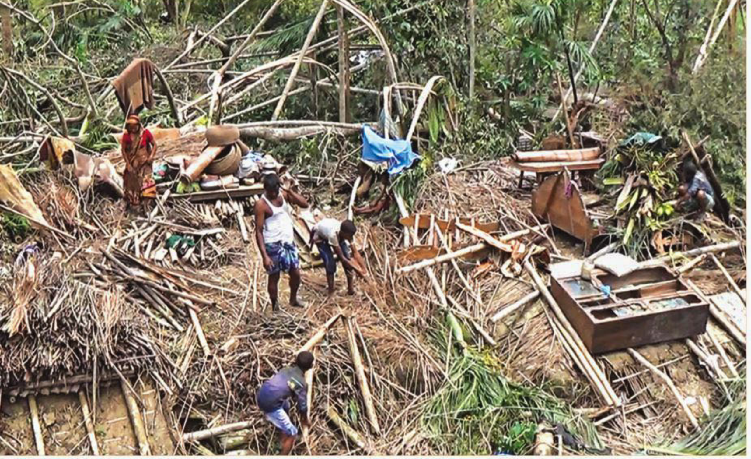
Devastated, a family gathers the remnants of whatever's left of their home in Jagannathpur village of Salukabad union in Bishambharpur upazila in Sunamganj after a nor'wester rampaged through many areas in the district early yesterday, damaging as many as 200 houses. A teenage girl was also killed and 50 others injured as a result of the storm. PHOTO: DWOHA CHOWDHURY
