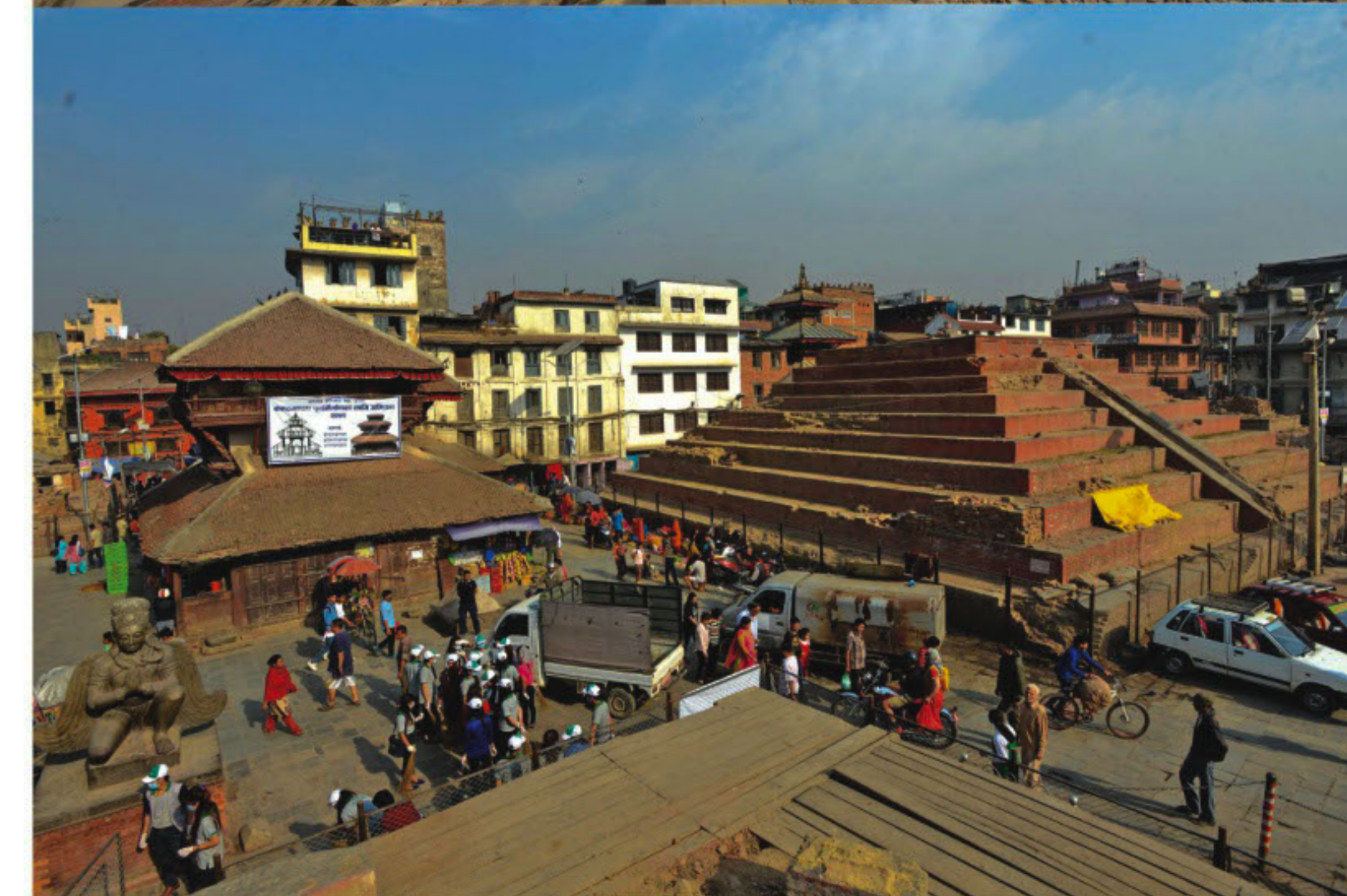
Photographs shows earthquake-damaged buildings in Durbar Square in Kathmandu on April 28, 2015 (top) and the same scene on April 23, 2016. PHOTO: AFP
