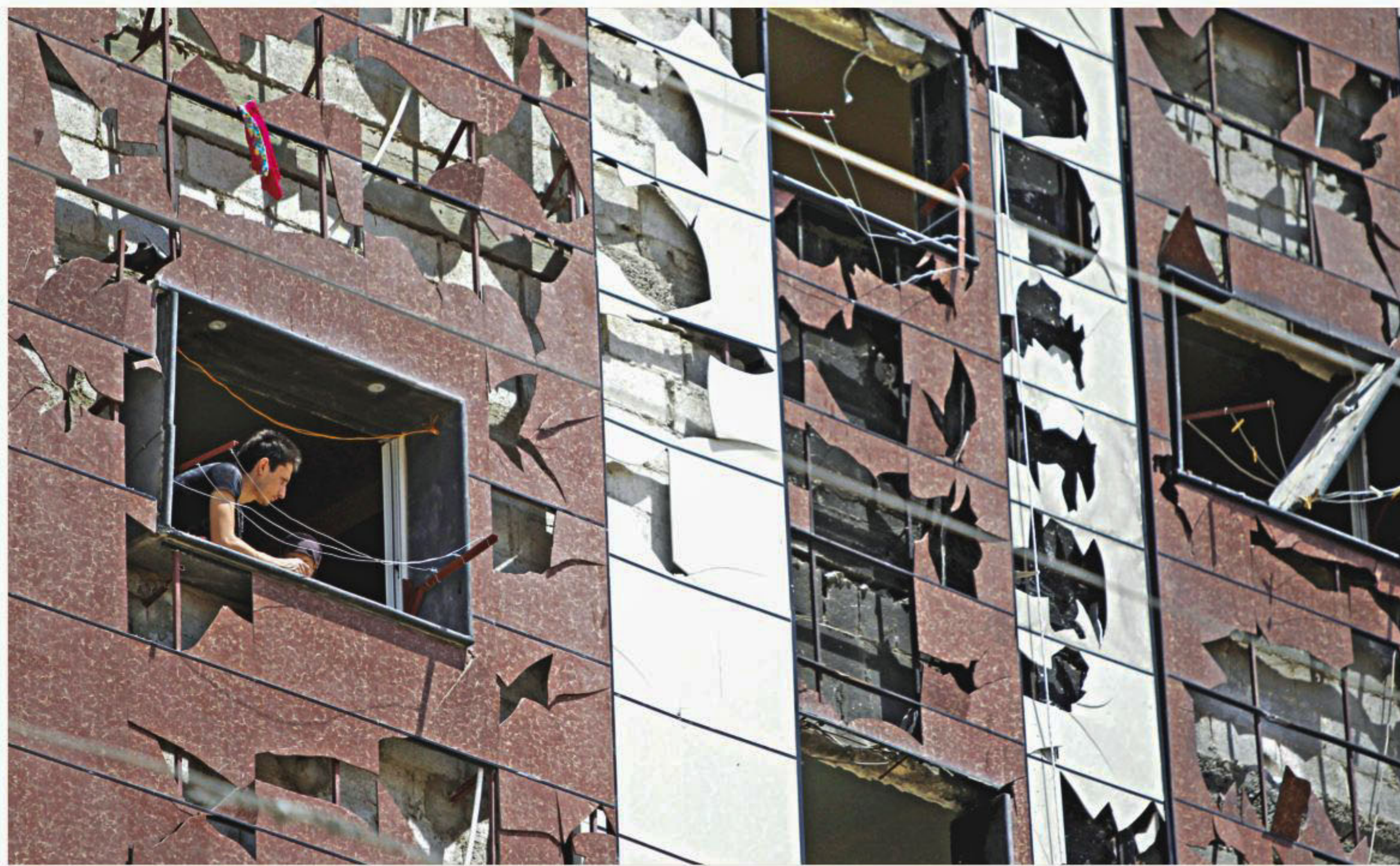
A civilian looks out from a window of a damaged building at the site of a car bomb blast near the revered Shia shrine of Sayyida Zeinab in Damascus, Syria yesterday. At least seven people were killed and twenty people wounded in the blast. The bomb struck Al-Diyabiyah, a town that serves as one of the gateways for the many pilgrims from around the world who visit the Shia holy site. PHOTO: REUTERS
