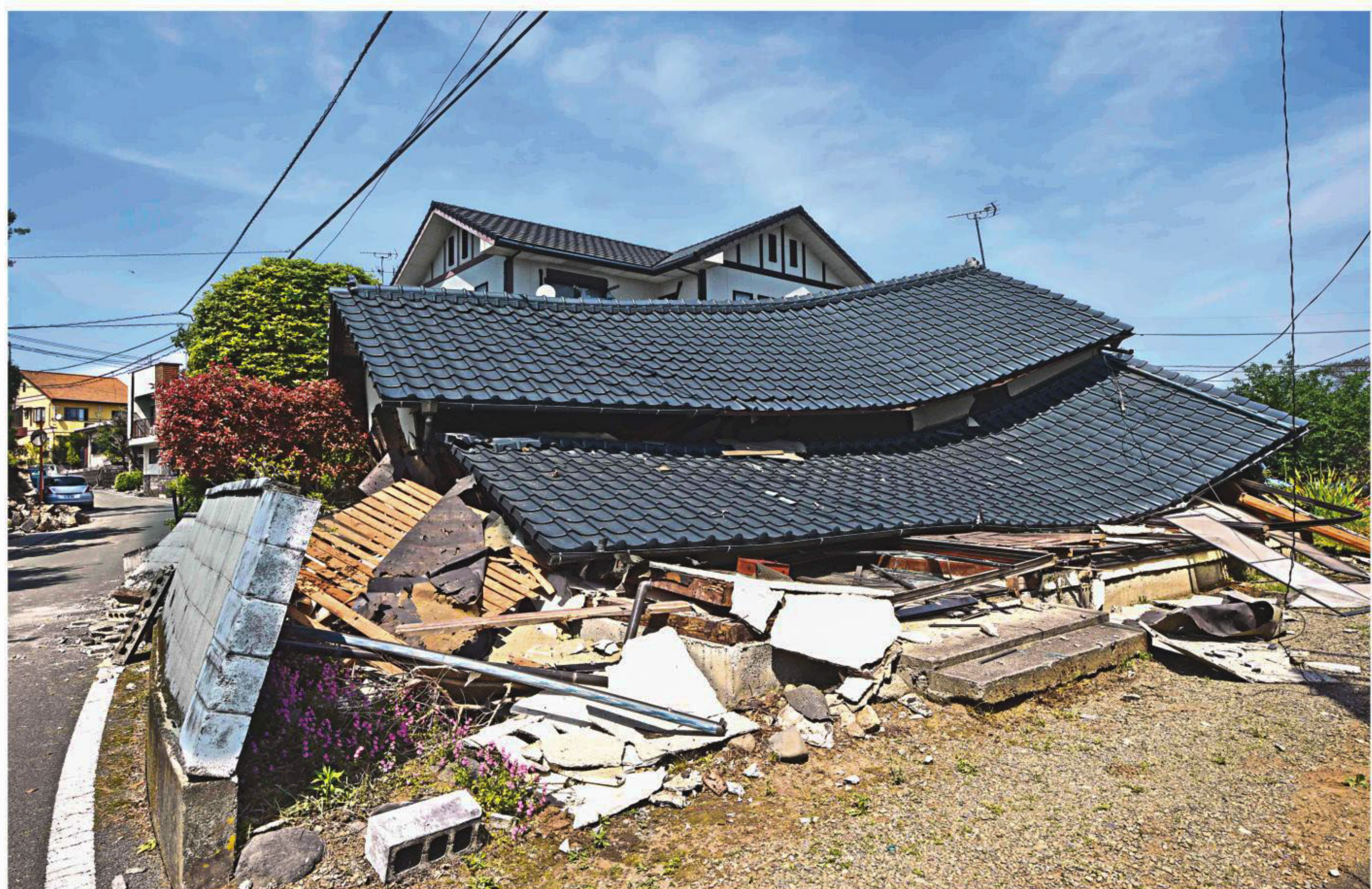
A quake damaged house in the town of Mashiki at Kumamoto prefecture in Kyushu Island yesterday. A strong 6.5-magnitude earthquake hit Japan's southwestern island of Kyushu on Thursday, demolishing homes and igniting fires.
