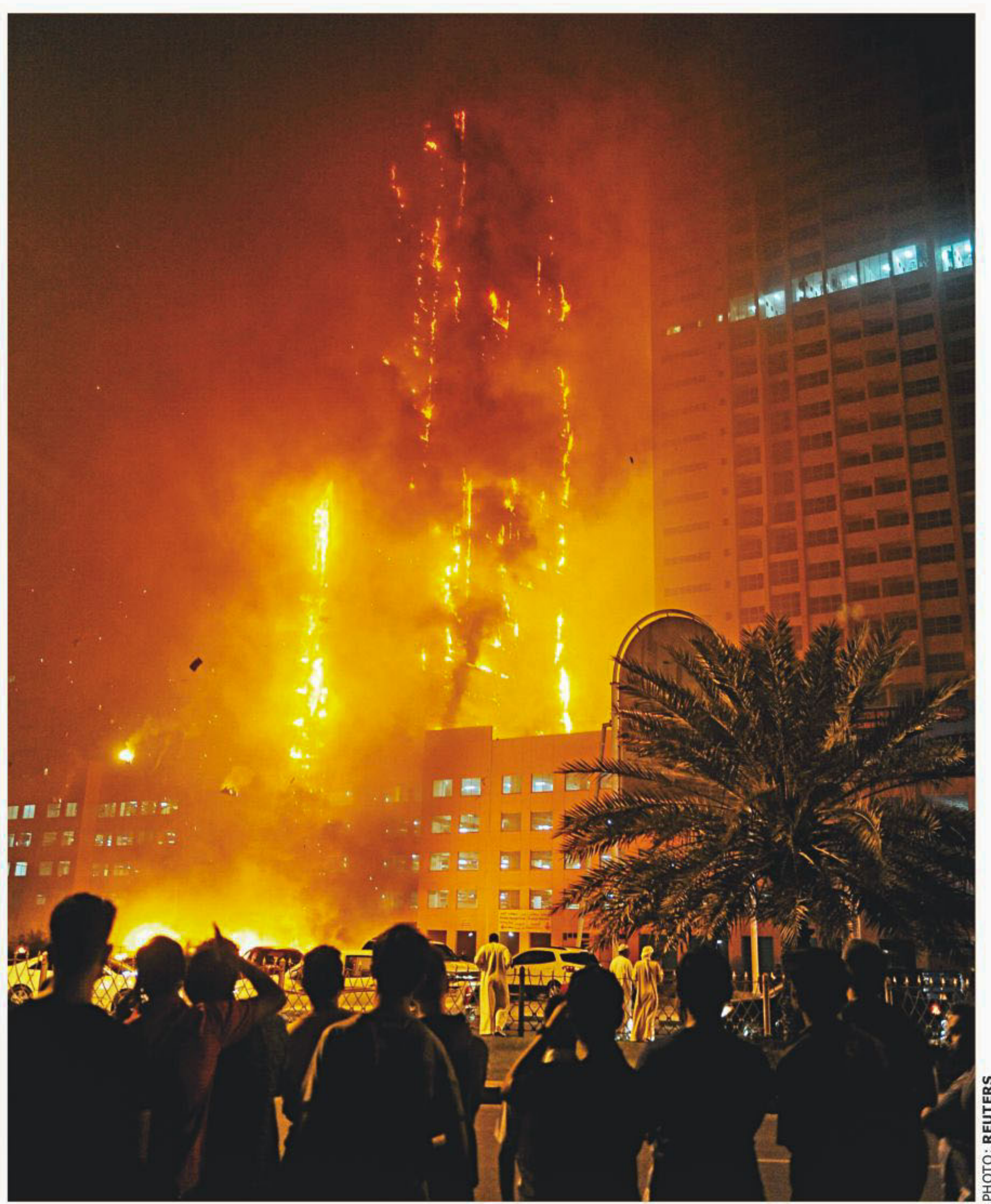
People gather after a fire broke out at a residential housing block in Ajman, UAE, yesterday. Firefighters brought the fire under control that broke out on Monday night, injuring five people. At least two towers of the 12-tower cluster were gutted. The cause of the fire was not immediately known.
