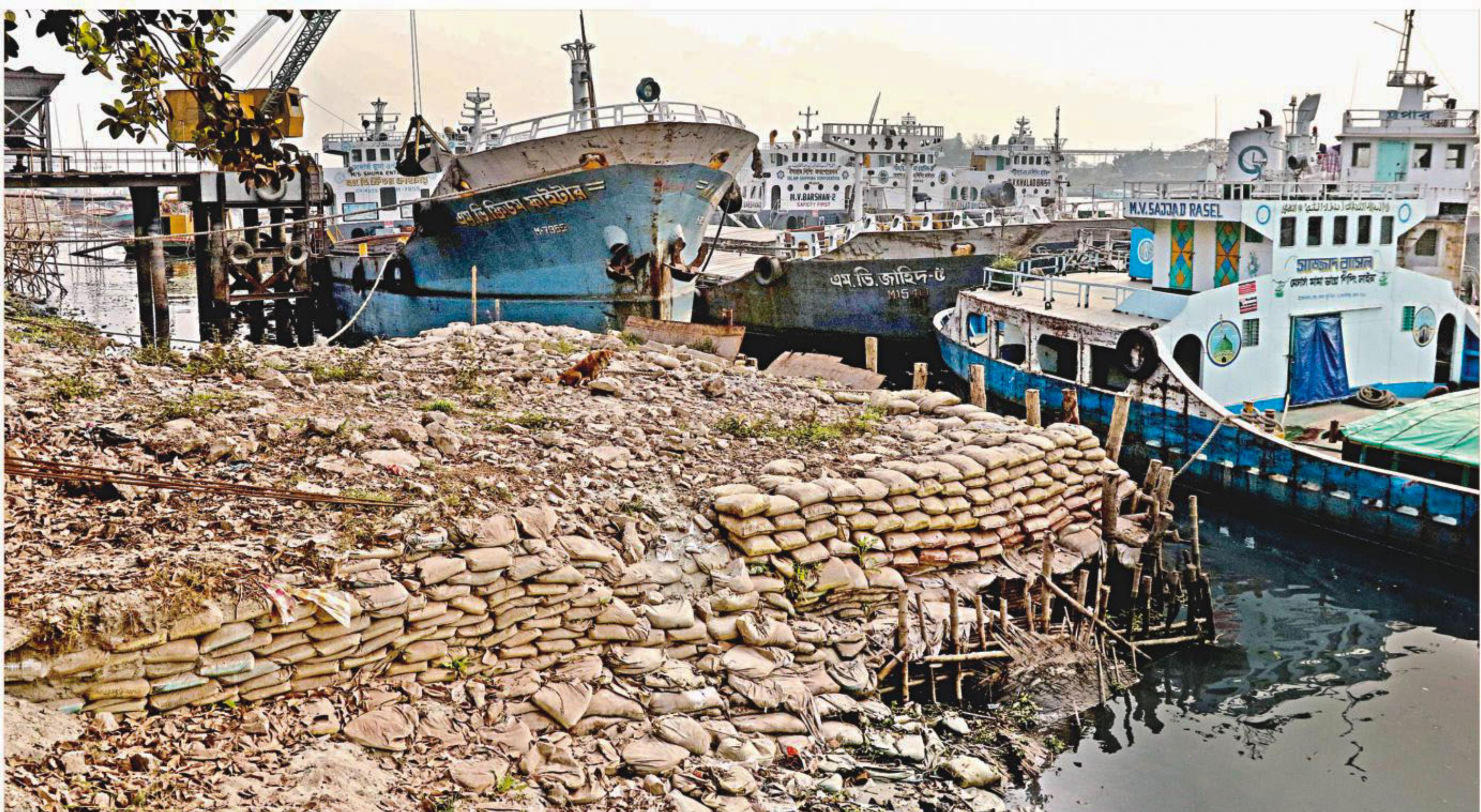
Unscrupulous businesspersons pile up sacks full of masonry on the bank of the Buriganga and extend those to 100 feet into the river at Shyampur in Narayanganj so that they can berth vessels and load and unload goods easily, narrowing down the water body. Three to four such berthing points were also set up in the area with Bangladesh Inland Water Transport Authority (BIWTA) turning a blind eye for nearly one and a half years. The photo was taken recently.
