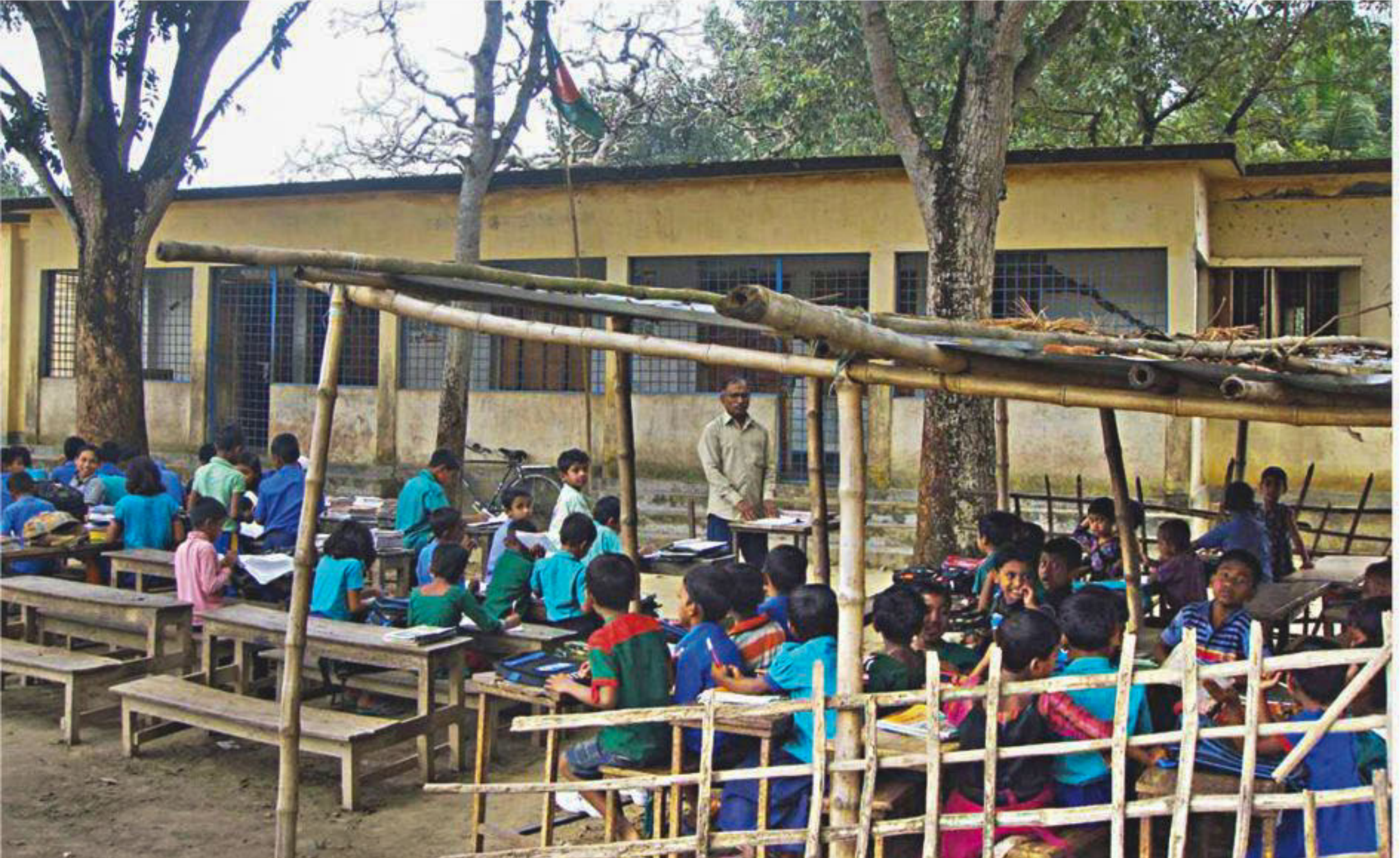
Students of Satura Government Primary School in Kotchandpur upazila under Jhenidah district attend classes under the open sky as their schoolhouse was declared abandoned three years ago.
