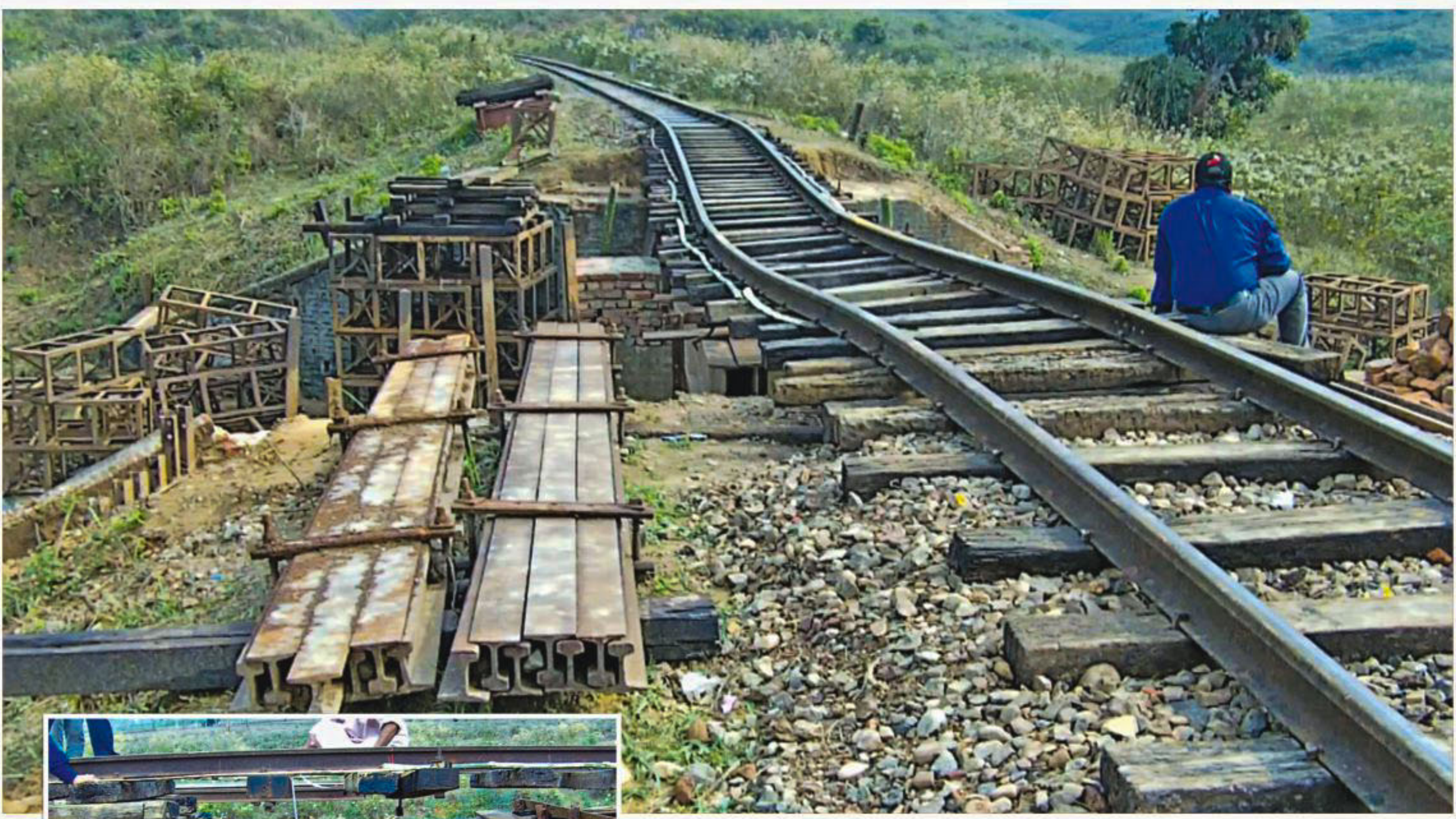
The warped portion of a rail track at Bhanugach in Sreemangal of Moulvibazar after heavy rain washed away the soil underneath, below. Rail communications between Sylhet and other parts of the country were suspended for around 14 hours since 3:00am yesterday as the track was unfit for train movement. Story on page 6.
