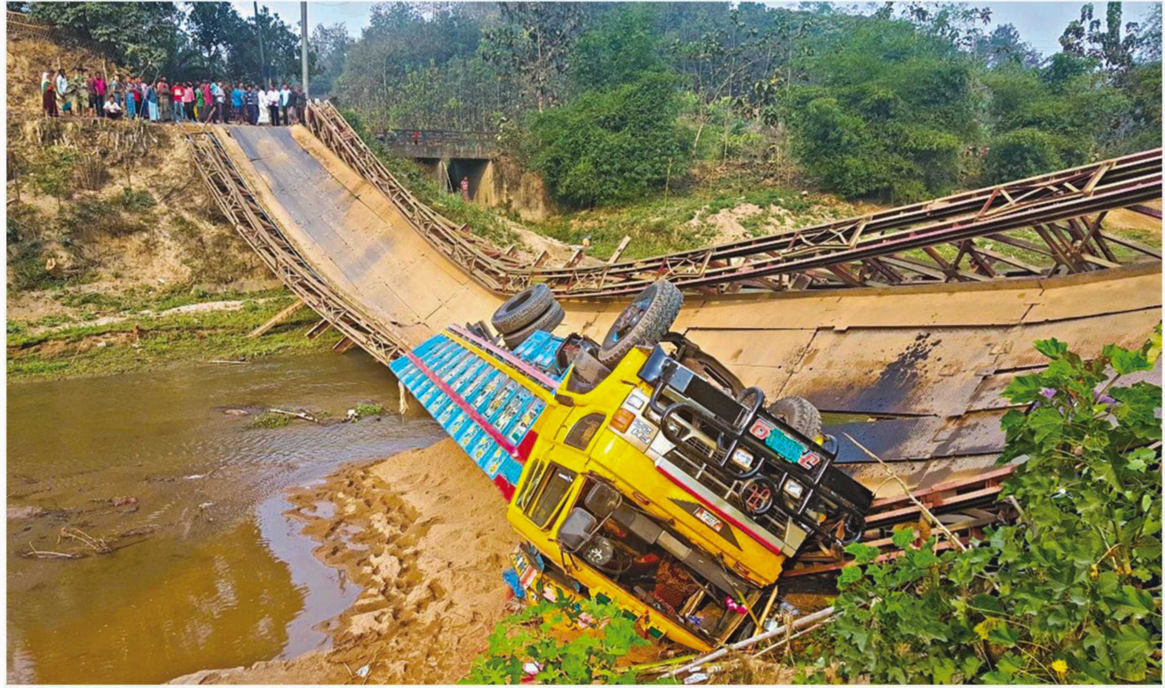
The Bailey bridge over Kansama Canal in Bandarban's Rowangchhari upazila collapsed under the weight of a truck "overloaded" with sand on Sunday, snapping road communications between the district town and the upazila. The 45-metre bridge had the capacity of vehicles weighing just five tonnes but trucks with heavier loads were using the bridge.
