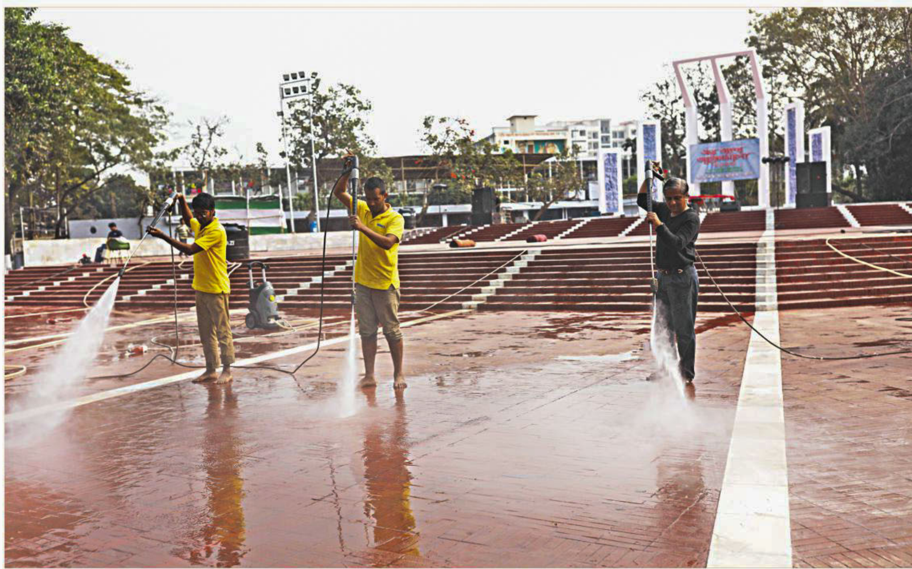
Central Shaheed Minar in the capital being hosed down with high pressured water yesterday and primed up for February 21 or Language Movement Day under a corporate social responsibility initiative of Greenland Technologies Limited, working on behalf of Dhaka University.
