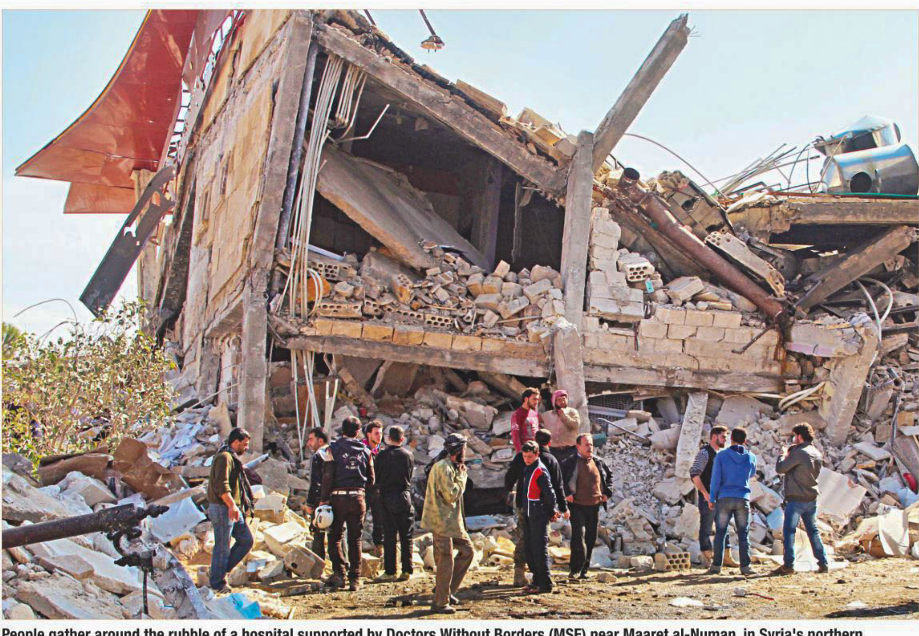
People gather around the rubble of a hospital supported by Doctors Without Borders (MSF) near Maaret al-Numan, in Syria's northern province of Idlib, yesterday, after the building was hit by suspected Russian air strikes. MSF confirmed in a statement that a hospital supported by the aid group in Idlib province was "destroyed in air strikes". PHOTO: AFP
