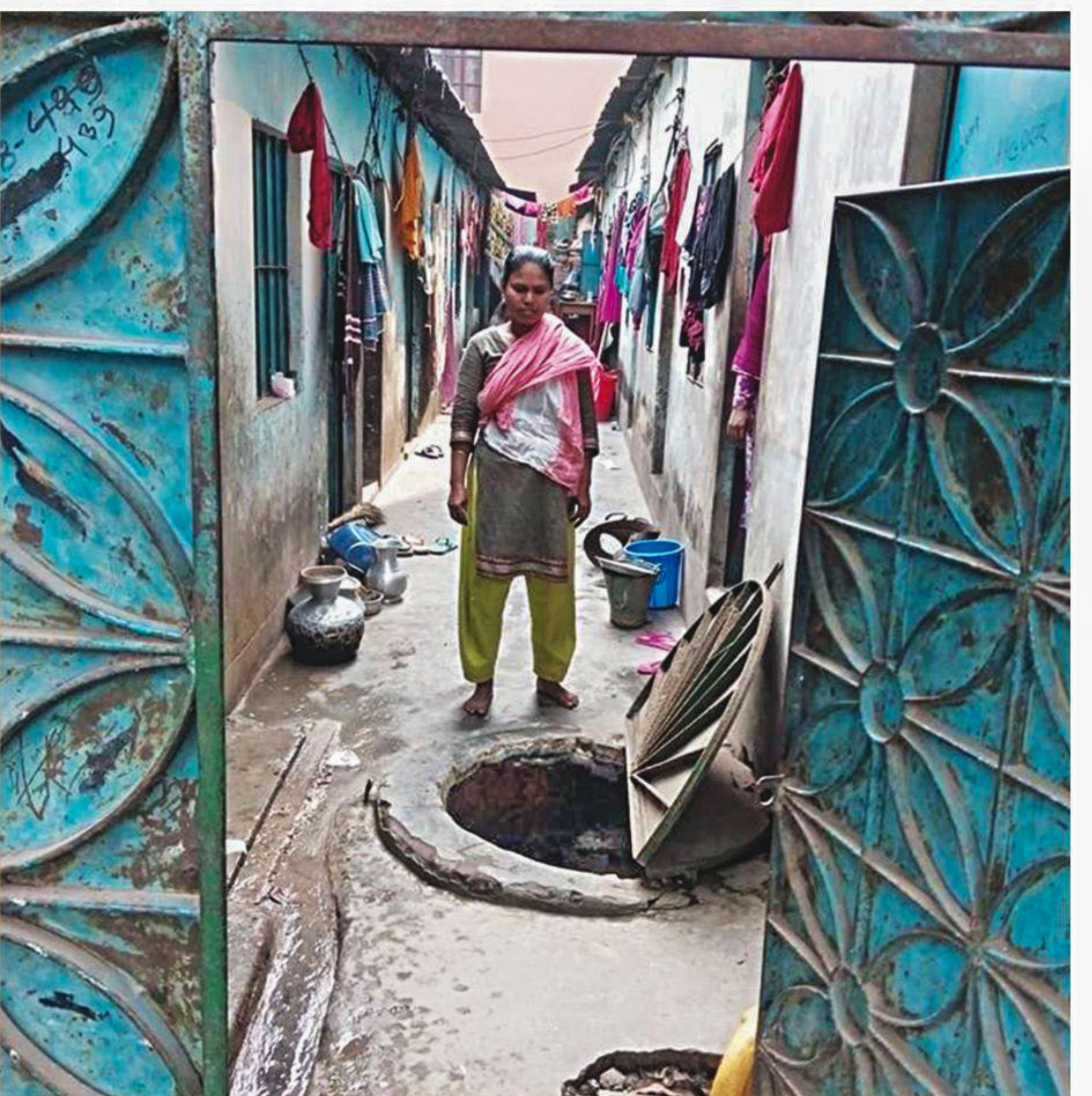
The lid of this underground water tank, around 12 feet in depth, is so heavy that families living in the adjoining 12 one-room tin-shed residences keep it open most of the time so as to make it easy to frequently access it. On why water is not being supplied directly to each residence to avoid the risk of a fall, especially by the many children living there, Rahima Begum, caretaker of this plot in Adarsha Nagar Lane 1, behind Kalshi graveyard, in the capital's Pallabi, could not provide a satisfactory answer. The photo was taken on Thursday.
