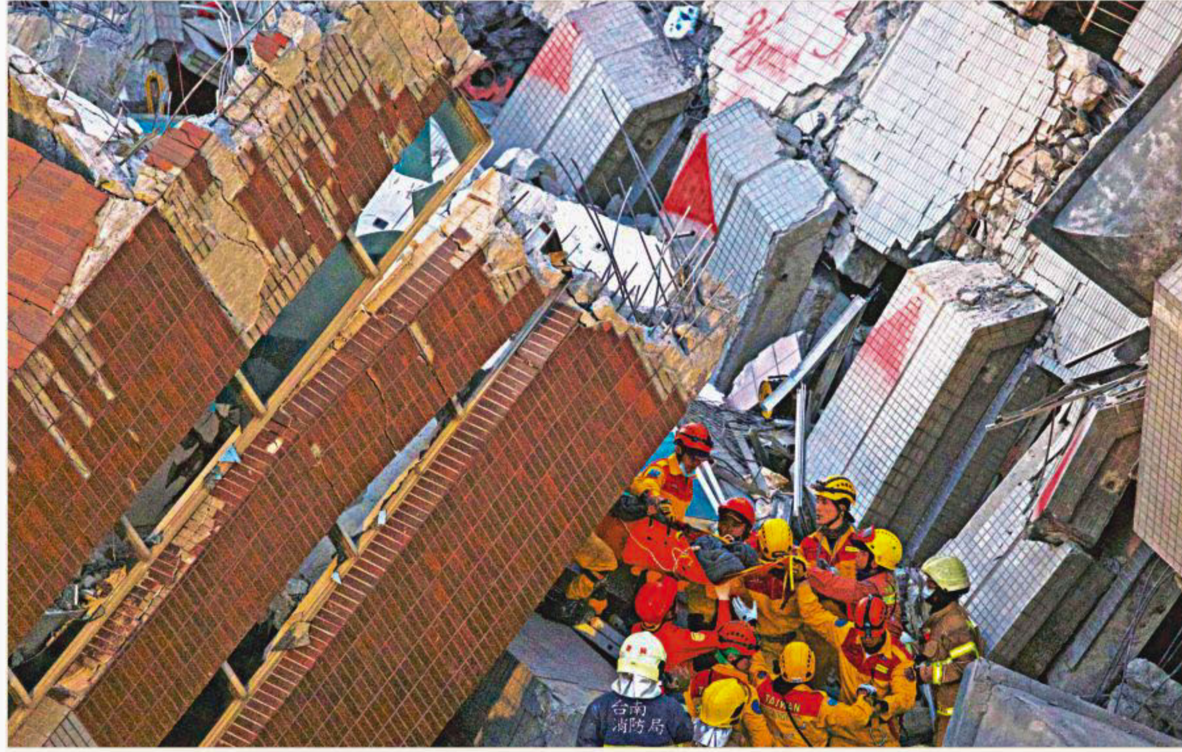
Rescuers carry a survivor out from the site where a 17-storey apartment building collapsed after an earthquake hit Tainan, southern Taiwan. Four more survivors were pulled alive from the rubble yesterday. The official death toll from the quake rose to 38, with more than 100 people missing.
