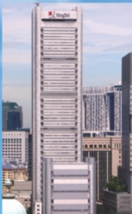
Telecom Building in Singapore
