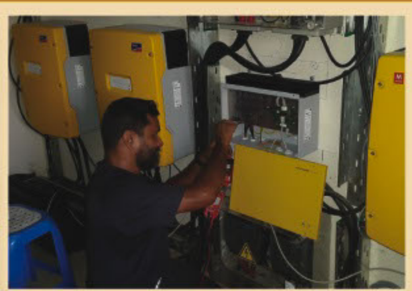
Commissioning of SEBL- 177 kWp project at Monpura, Bhola
