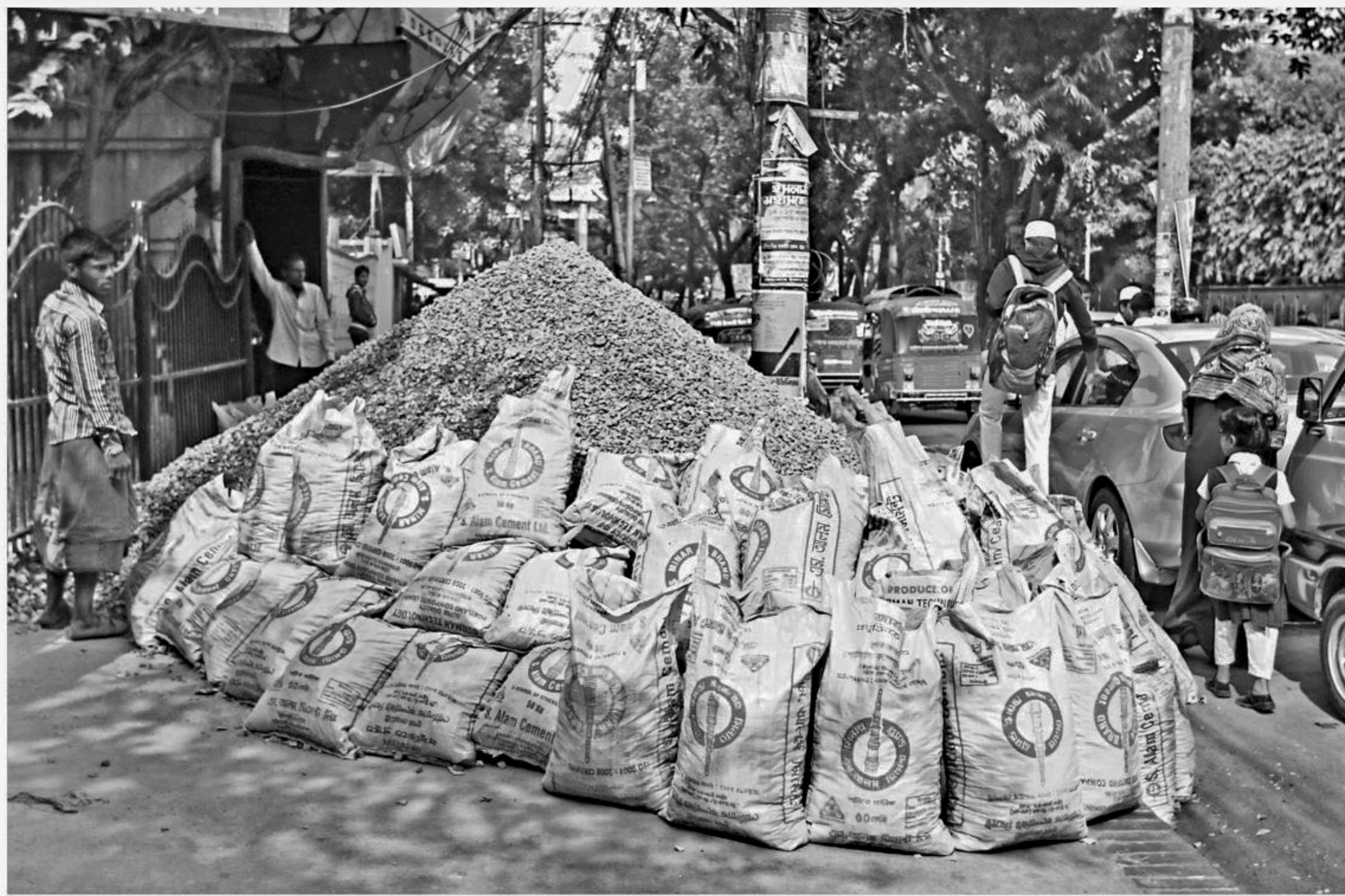
Construction materials of an adjoining building block this footpath in front of Chittagong Press Club while undesignated parking takes up space on the adjacent Jamal Khan Road in the port city yesterday although both practices have been banned by the city corporation.
