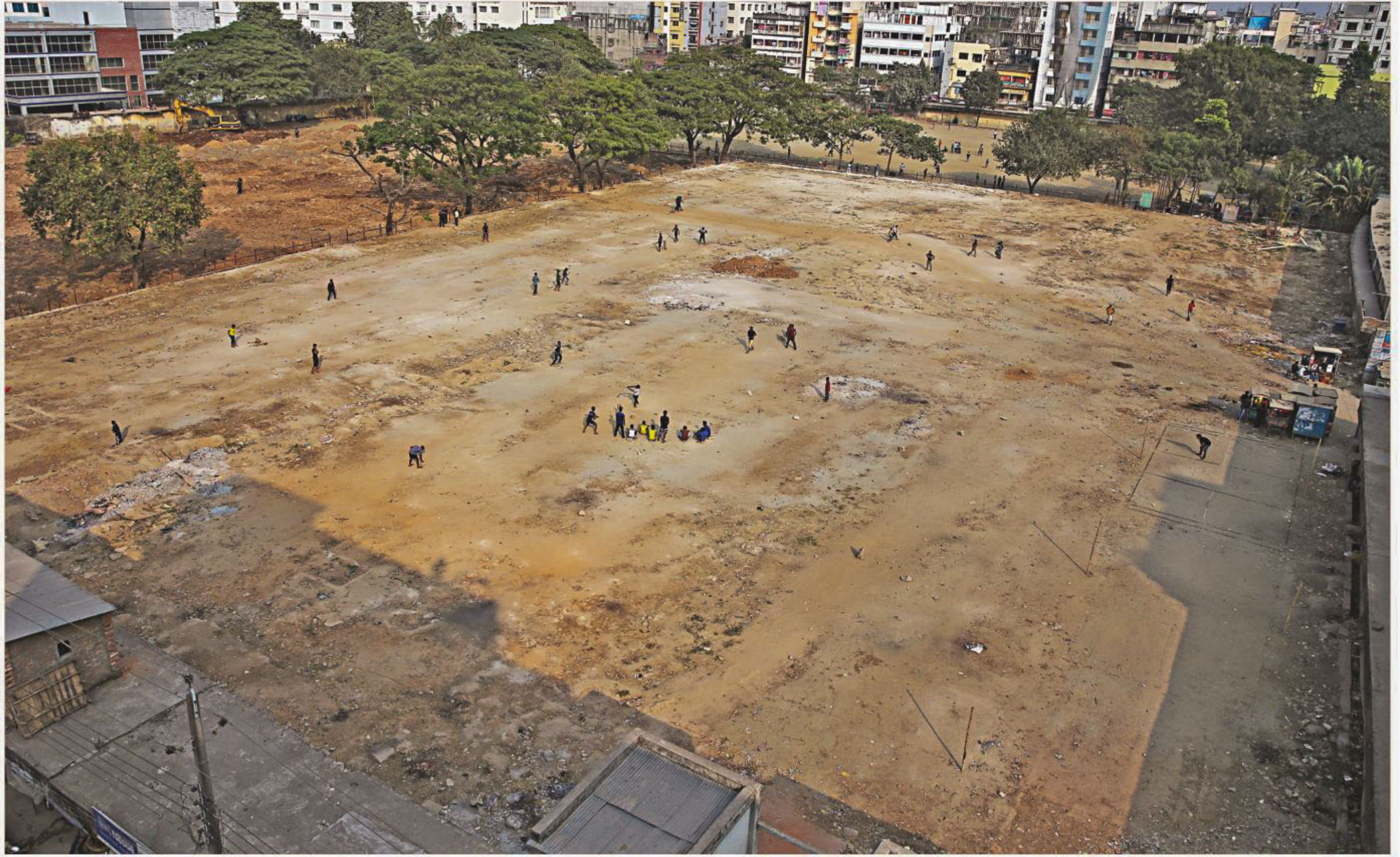
The part of the enormous Dhupkhola Math, which is open to all, has not been repaired by Dhaka South City Corporation (DSCC) after its surface was badly damaged for storing construction materials of Mayor Mohammad Hanif Flyover. However, defying risks of injury in the field riddled with craters and littered with masonry, children have started coming to play there. The photo was taken yesterday.
