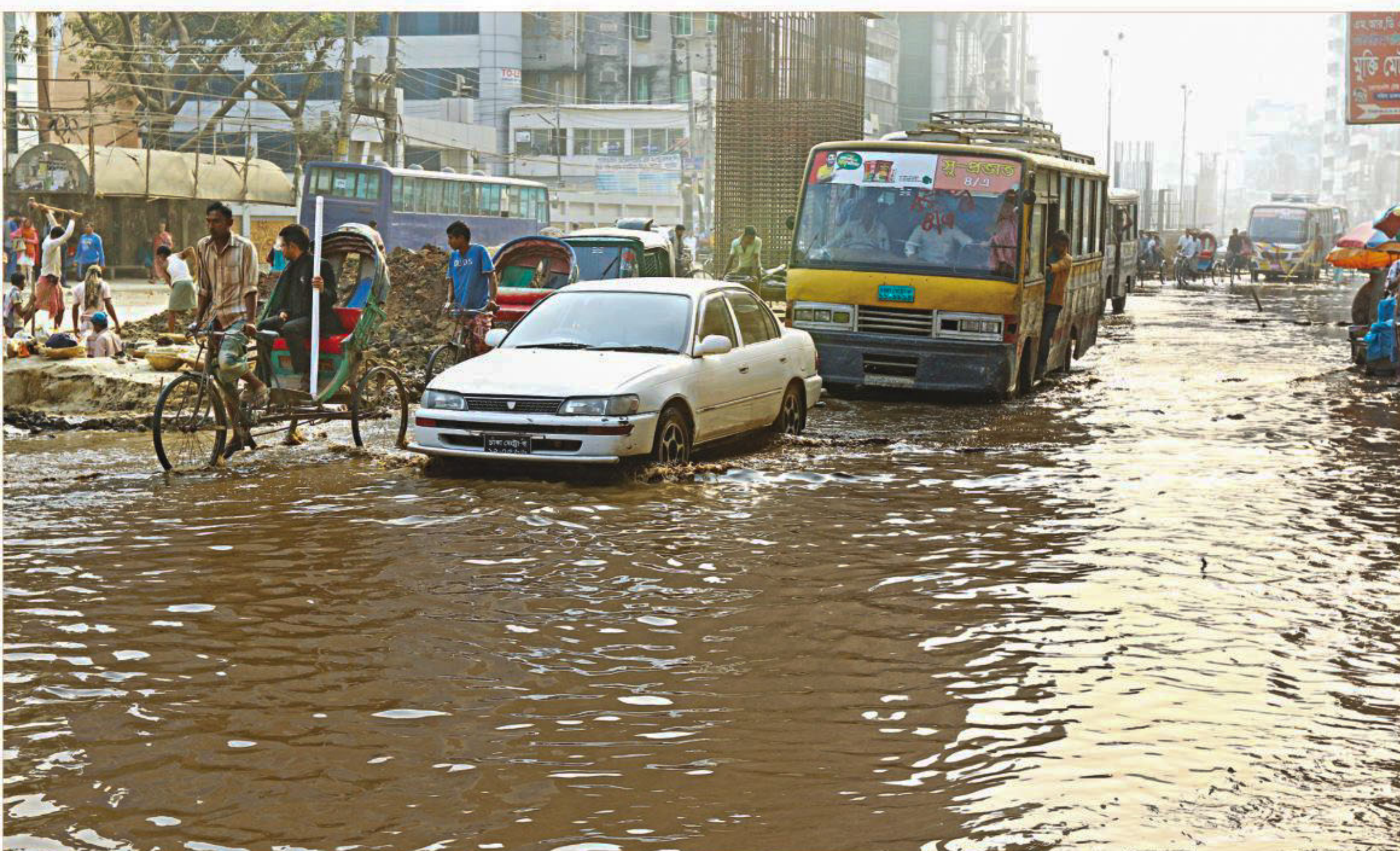
Though reminiscent of the rainy season, the water collecting here on Siddheswari Circular Road near the Malibagh intersection in the capital originated from sewers and construction works of the Malibagh-Moghbarz flyover project, causing sufferings to those who have to use the road. The photo was taken yesterday.
