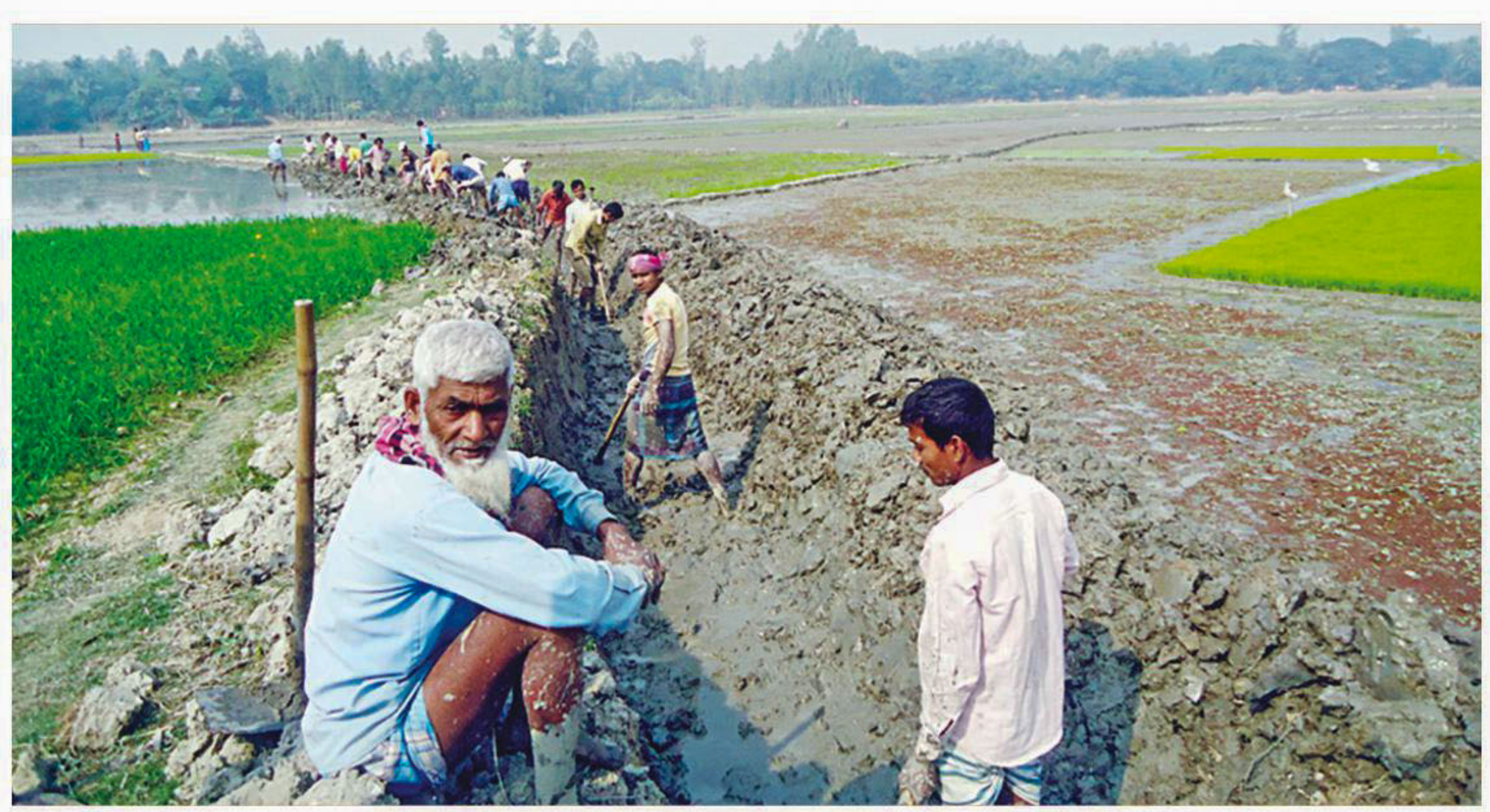
Villagers dig an irrigation canal across a vast farmland in Manda upazila of Naogaon. The canal, measuring 10 feet wide and 3km long, was dug by more than 50 local residents after their appeal to the government authorities for excavation went in vain. This irrigation channel is expected to boost the agricultural output from the land. The photo was taken Tuesday.
