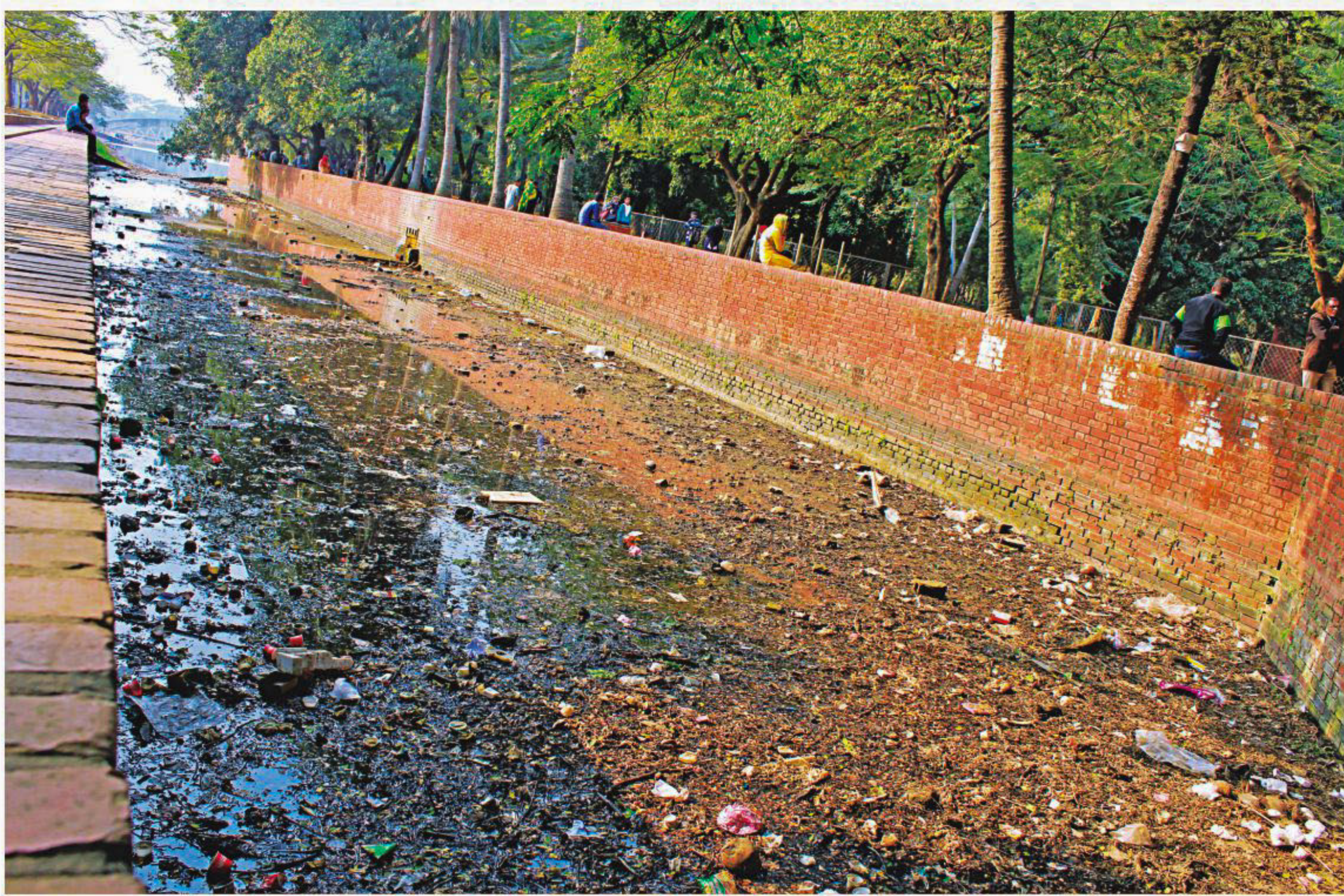
Garbage fills a part of Crescent Lake in Chandrima Udyan. The lake was built for enhancement of the beauty of the sprawling Jatiya Sangsad Bhaban complex but it is doing the opposite now due to lack of care. The photo was taken last week. PHOTO: MD KAWSAR
