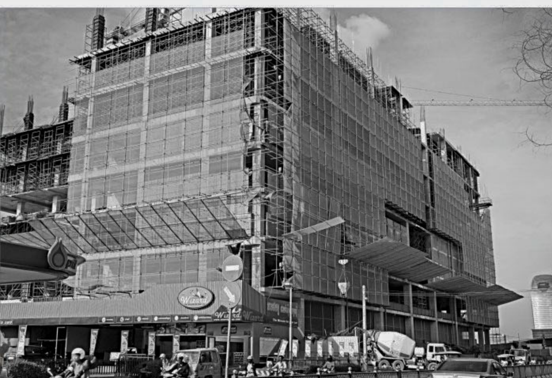
A building is under construction in Phnom Penh, Cambodia.
