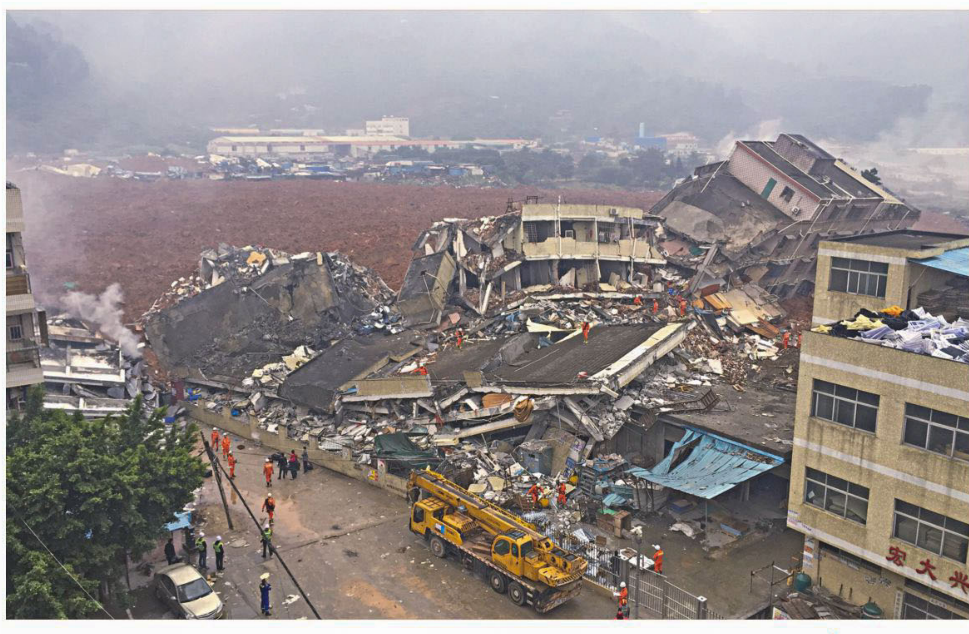
Damaged buildings are seen as rescuers search for survivors in an industrial park in Shenzhen, Guangdong province, China yesterday. A massive landslide at the park buried 22 buildings and left 41 people missing.
