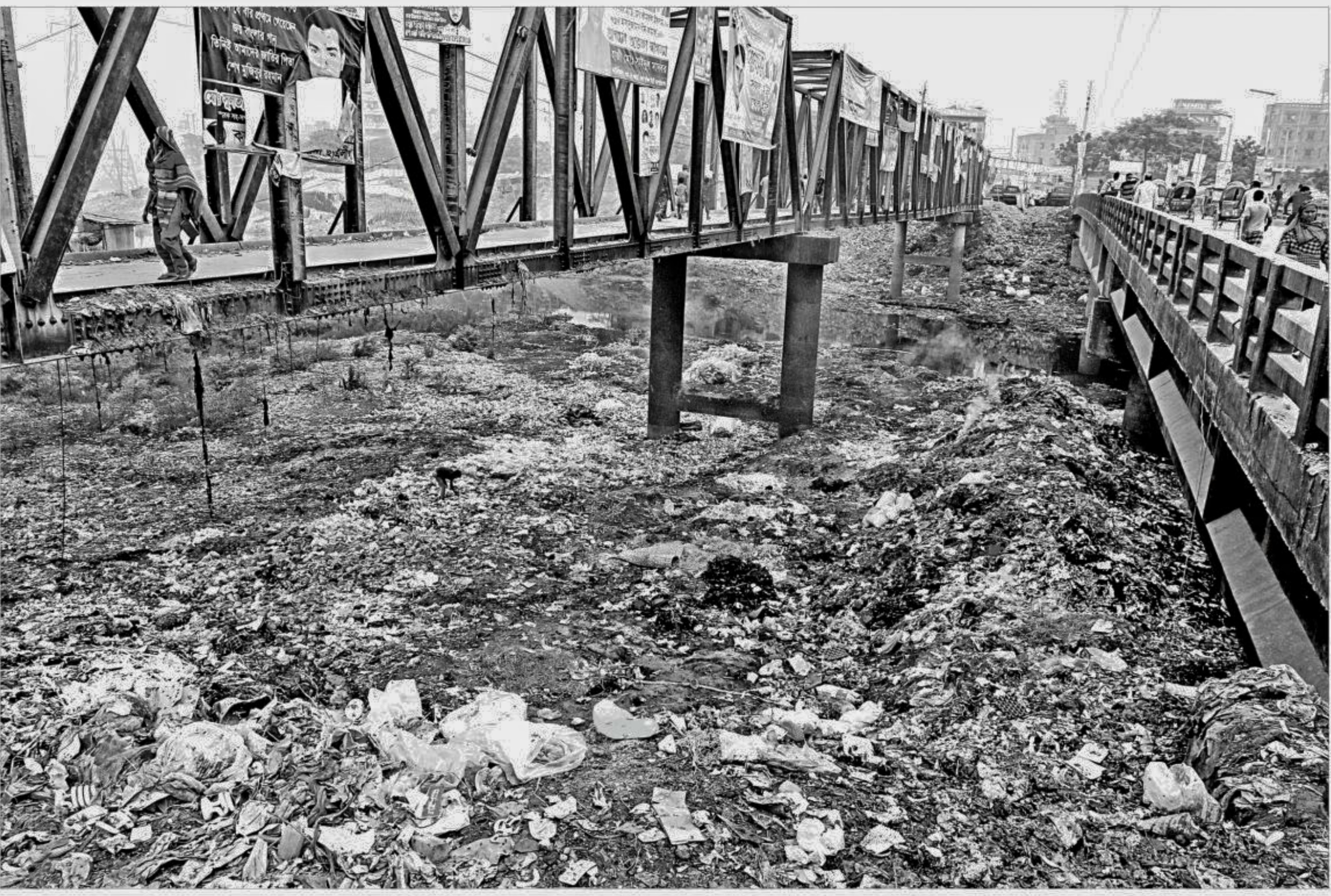
Unabated dumping of garbage has choked off this channel of the Buriganga river under the bridges leading to Kamrangirchar from Lalbagh in the capital. The photo was taken yesterday. PHOTO: ANISUR RAHMAN
