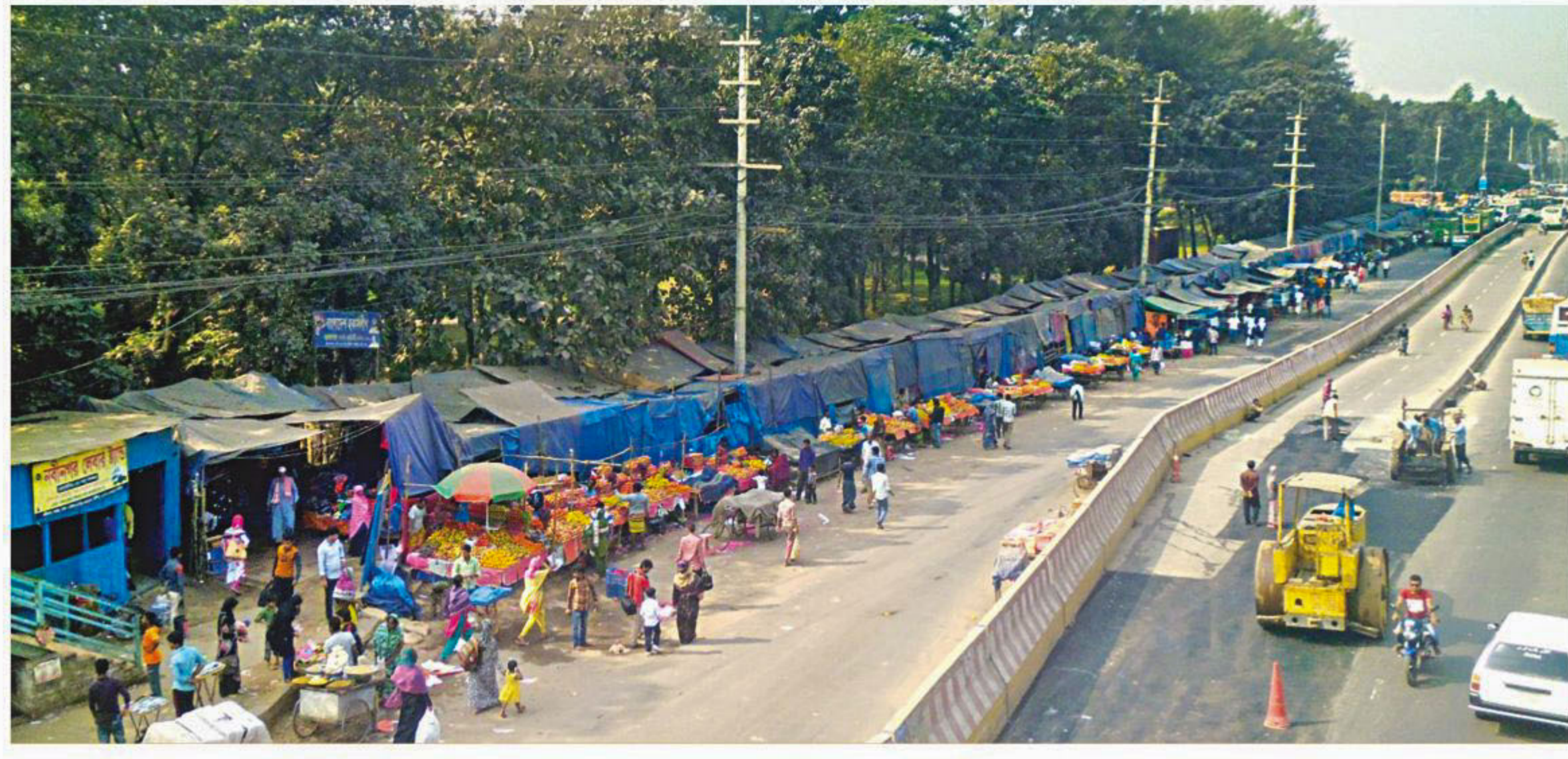
Illegal shops lining the south-western edge of the National Memorial complex in Savar, outside the capital, hide the beauty of its vast premises. Though the structures are removed twice a year, the traders set those up again with support from powerful men. The photo was taken Tuesday. PHOTO: RASHAD AHAMAD
