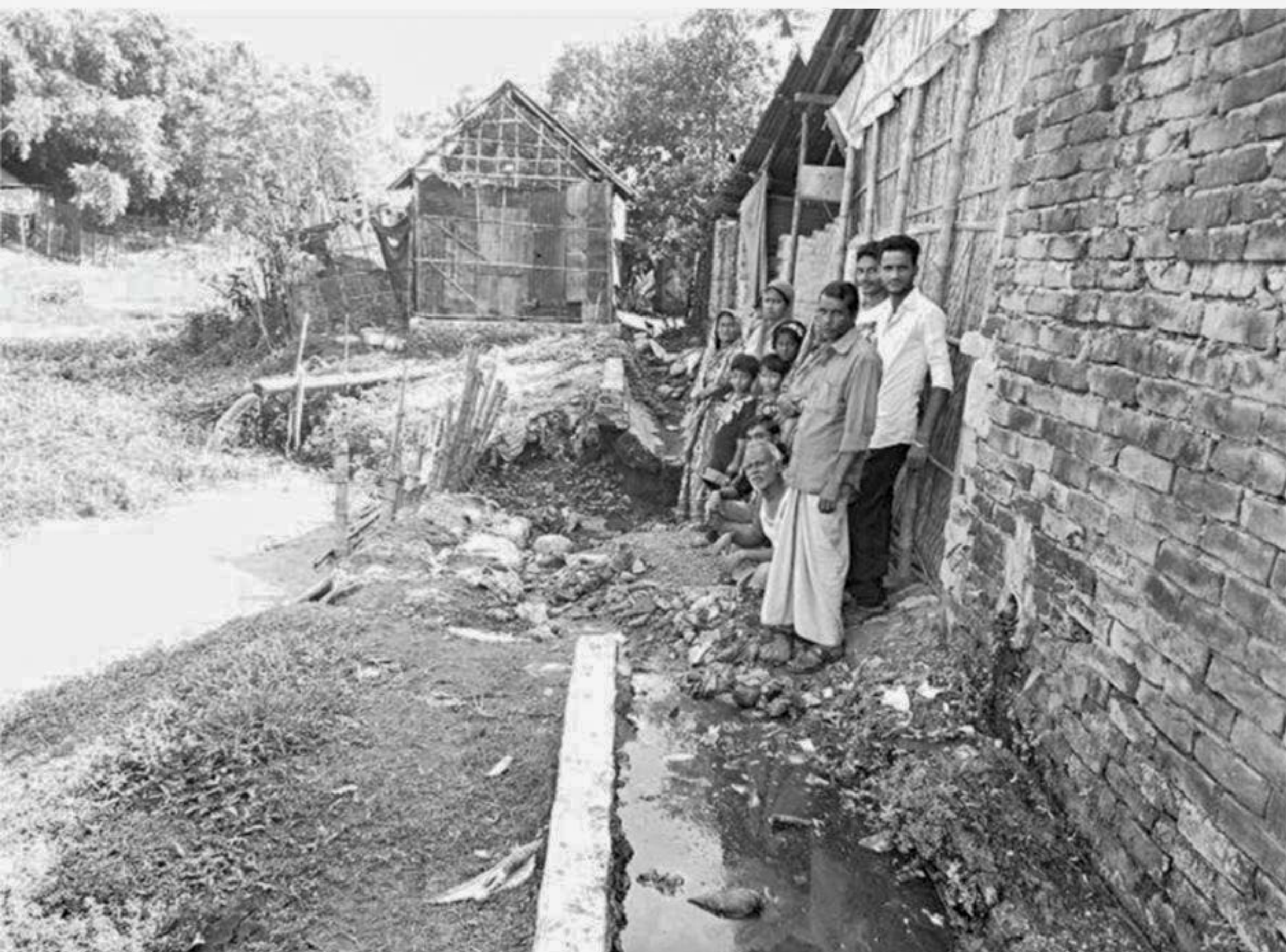
PHOTO: STAR Sand extraction from 30 to 40 feet depth of a pond, consequent creation of vacuum and collapse of this surface drain at Munshipara in Saidpur municipality in Nilphamari district led to pollution of underground water, causing tube-wells in the area to draw dirty and unusable water.
