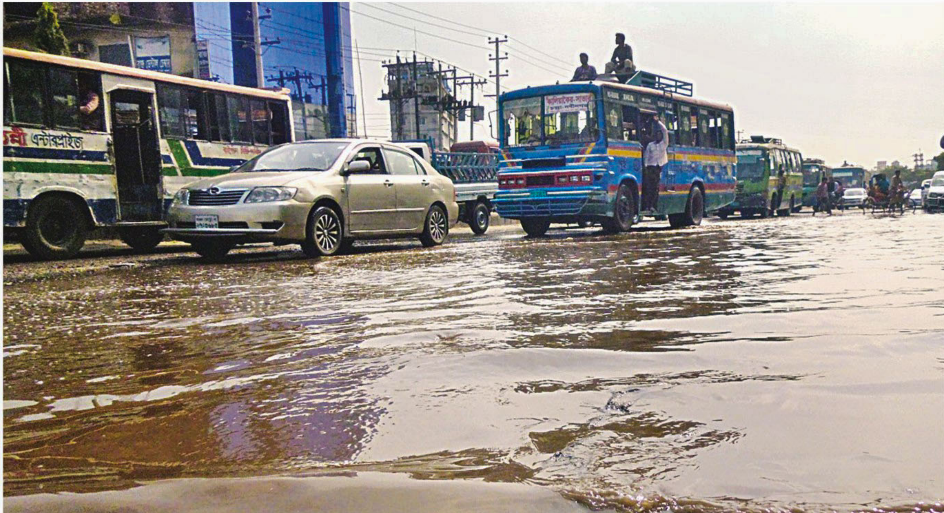
The Dhaka-Aricha highway at Savar Bus Stand is flooded with sewage due to very poor drainage. The sewage used to pass in drains that go through a state-run horticulture centre there. However, the centre blocked the drains as sewage always spilled over killing their trees. The photo was taken yesterday. PHOTO: RASHAD AHAMAD
