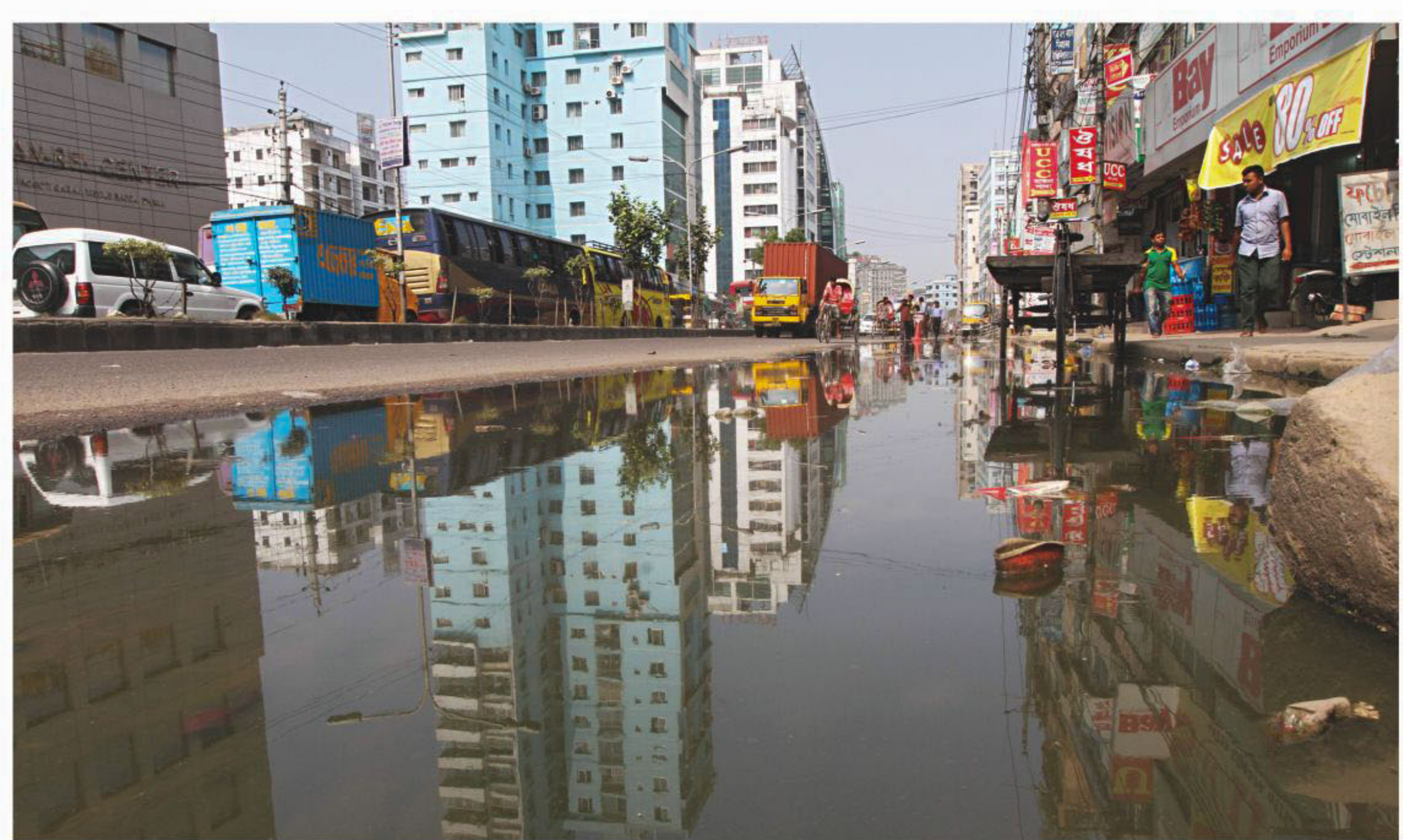
Dhaka city does not need a spell of rain to have its streets waterlogged. In different parts, sewerage water stays on the road round the year because of broken underground pipes or the absence of a proper drainage system. The photo was taken at Madhya Badda on Progoti Sarani yesterday.
