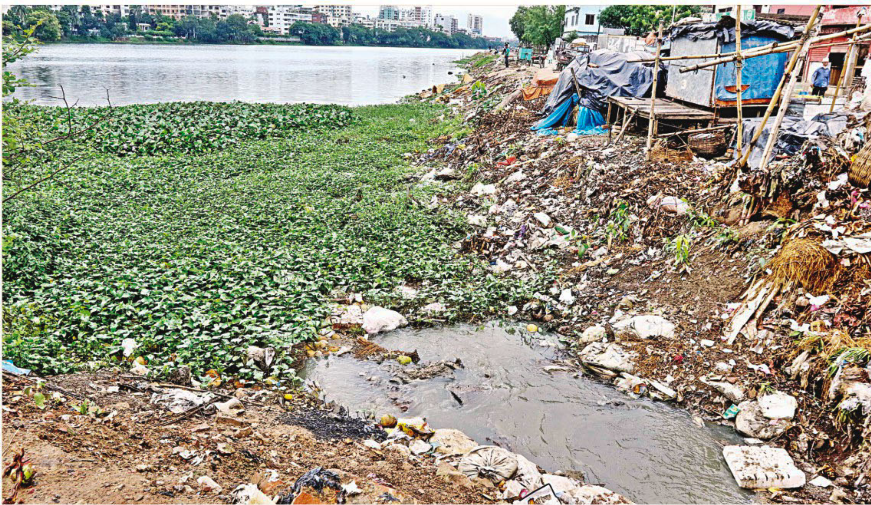
Sewage flows into Gulshan-1 Lake of the capital while garbage fills its bank but the authorities are as unperturbed as before about the pollution of the water body and ruination of its beauty. The Daily Star published photos of the lake several times before. This one was taken last week.
