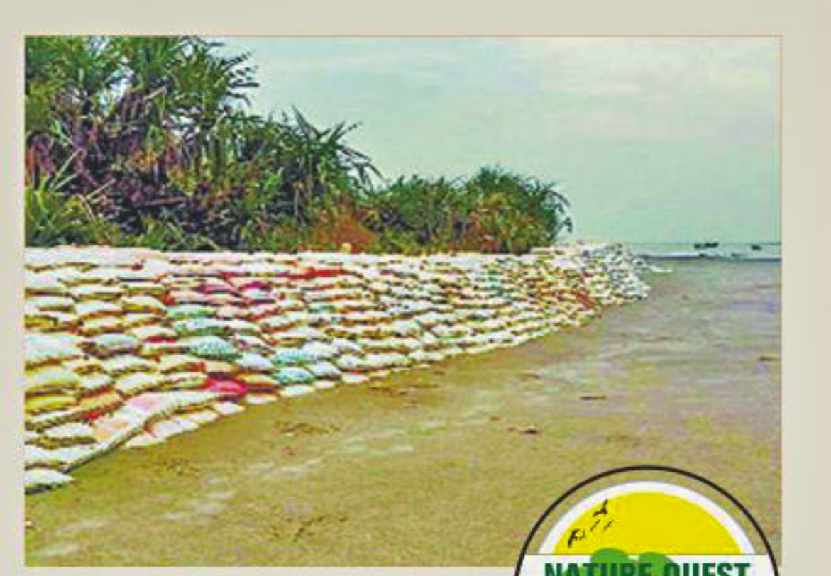
Sacks of sand piled up on the shore of the Bay at St Martin's Island to protect it from tidal surge.
