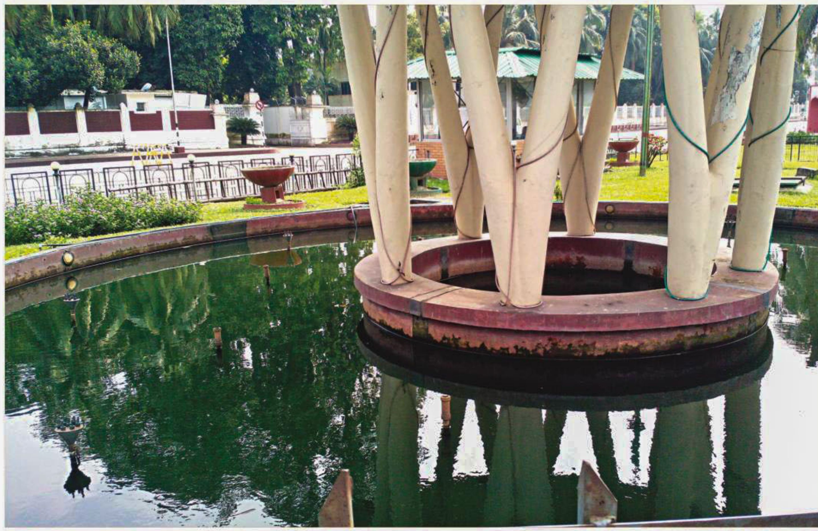
While the city dwellers are exposed to the mosquito-borne dengue fever, the fountain in front of Bangabhaban, the president's residence and the highest office of the country, has turned into a breeding ground of mosquitoes. This simply reveals how nonchalant the authorities are to the public health hazards. Requesting anonymity, a traffic constable said the fountain remained non-operational for the last several days. When contacted, the city corporation officials said they changed the water every one or two months but there was no way mosquitoes would breed there because the fountain was operated twice a day.
