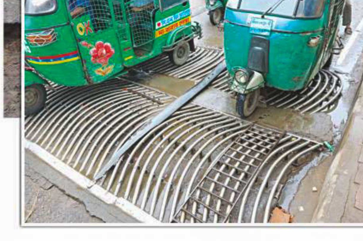
Bars installed on a street in Hatirjheel project area to prevent non-motorised vehicles from using the street have become a trap for motorbikes. Locals claimed that they welded a metal frame over the bars so that motorbikes could pass. Motorists complained that their vehicles lose traction going over the bars which sometimes cause traffic mishaps. PHOTO: ANISUR RAHMAN
