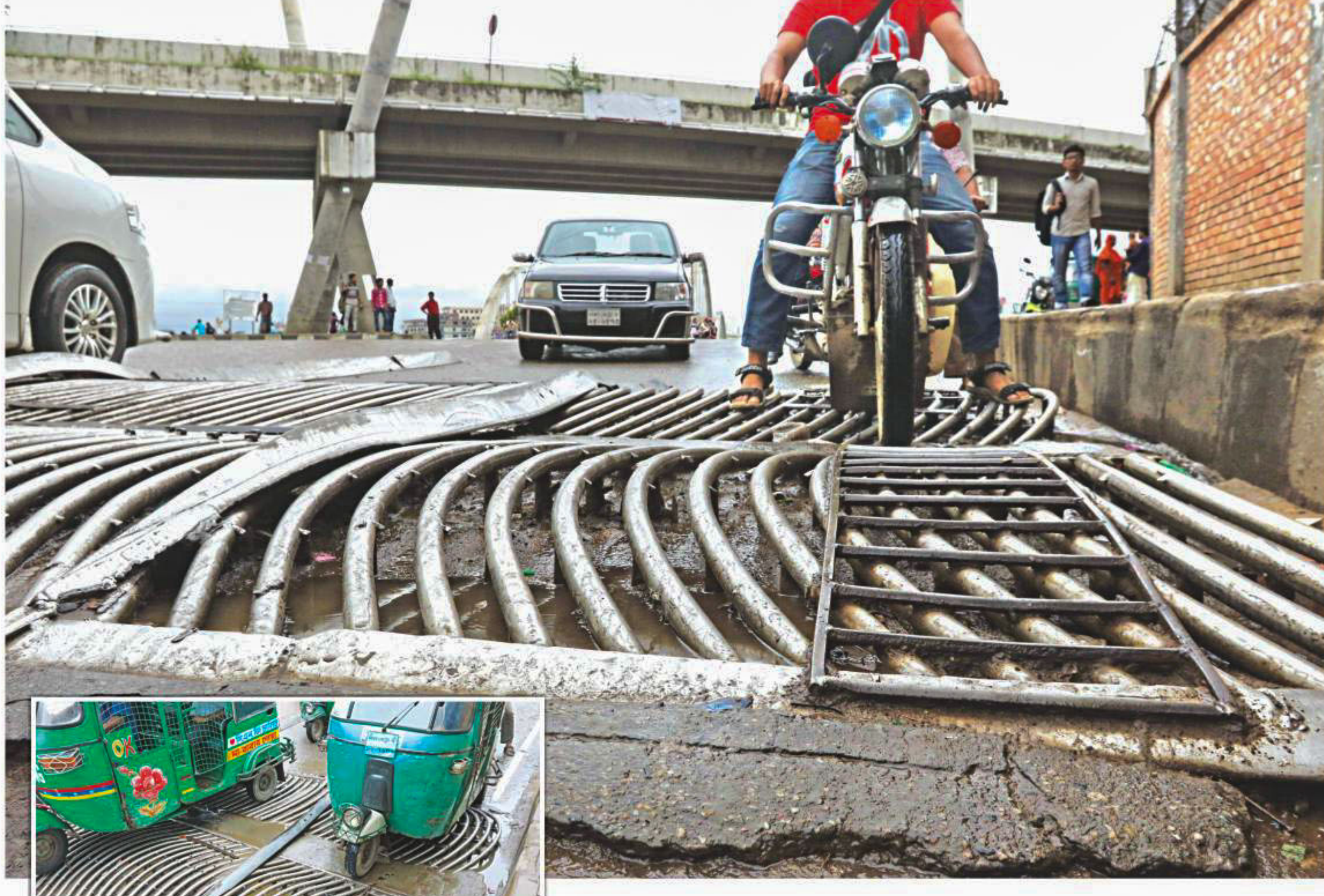
Bars installed on a street in Hatirjheel project area to prevent non-motorised vehicles from using the street have become a trap for motorbikes. Locals claimed that they welded a metal frame over the bars so that motorbikes could pass. Motorists complained that their vehicles lose traction going over the bars which sometimes cause traffic mishaps. PHOTO: ANISUR RAHMAN
