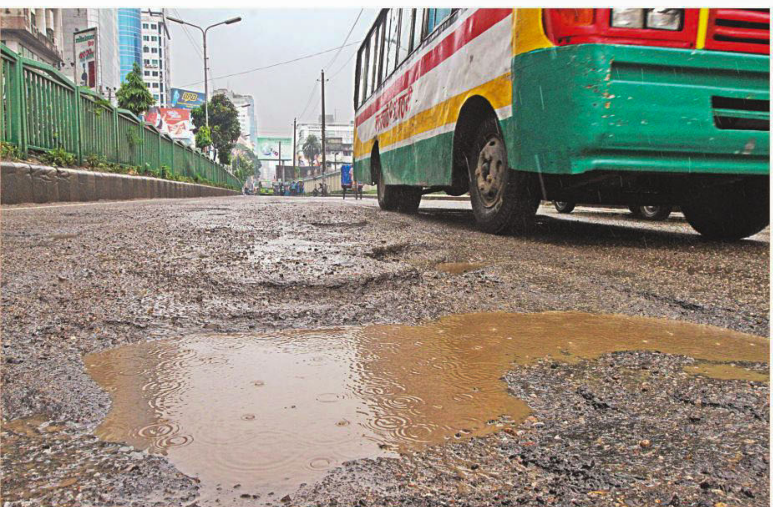
Potholes riddle Topkhana road in the capital with the recent rains worsening the condition. The photo was taken on Tuesday.
