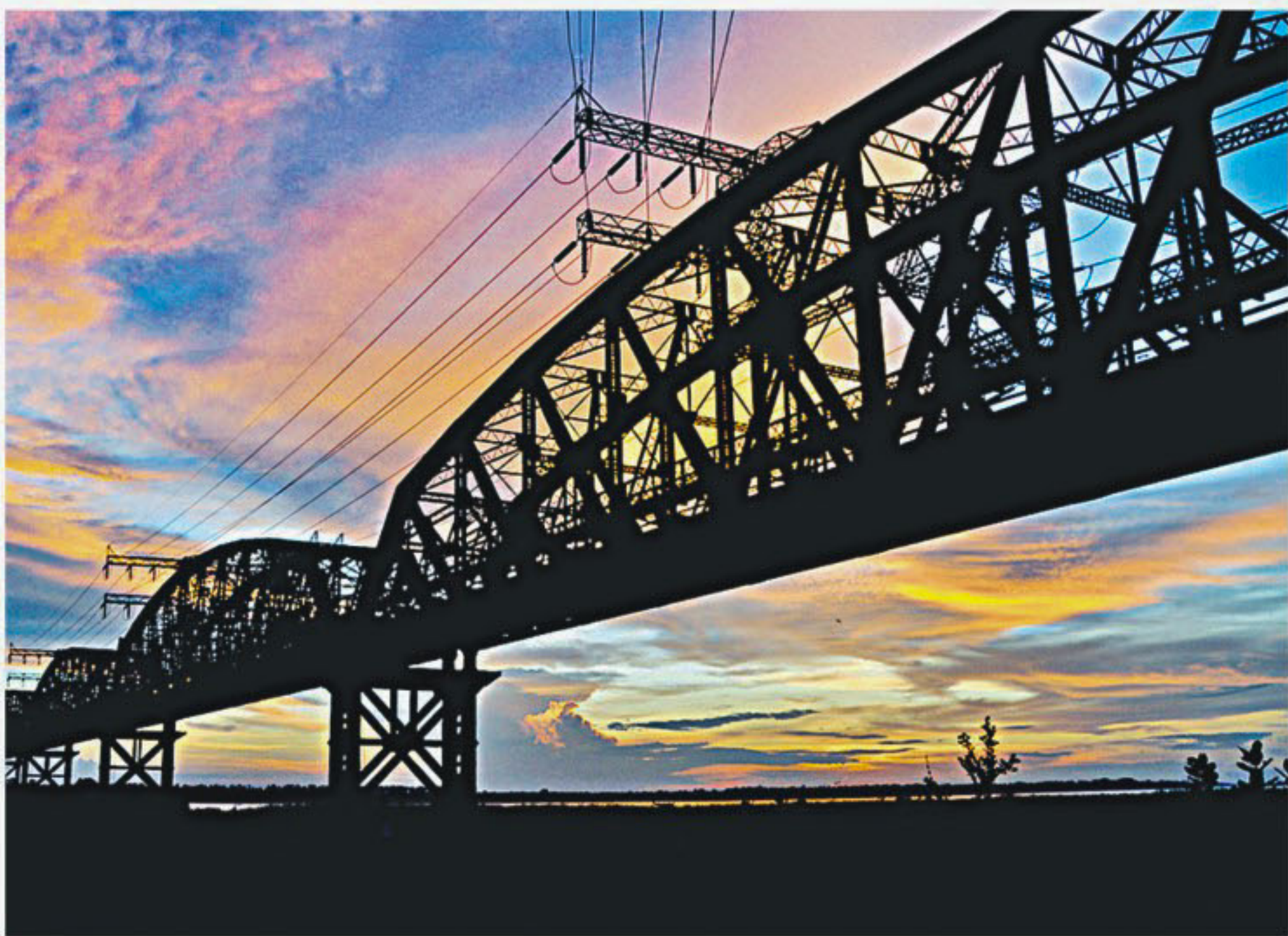
Hardinge Bridge on Padma located at Paksey.
