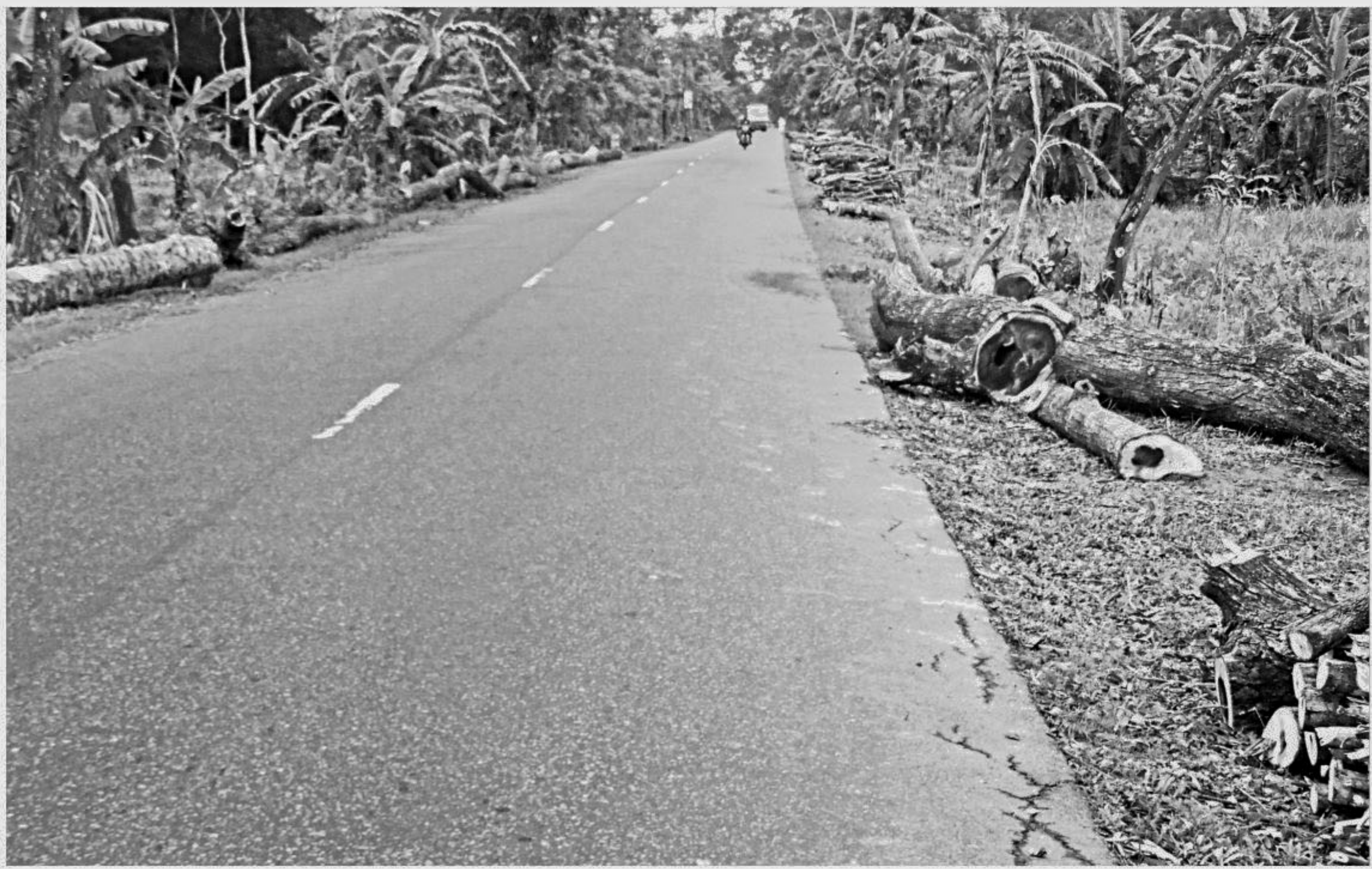
All the trees on the both sides of Barisal-Khulna highway from Shatpakia to Sutoriali in Nalchhity of Jhalakathi felled down in last one month after the forests department had floated a tender two months ago, saying that those became old enough. The department, however, started planting new trees there. Green experts said the tree felling will cause environmental degradation for a period of time. The photo was taken at Shatpakia yesterday.
