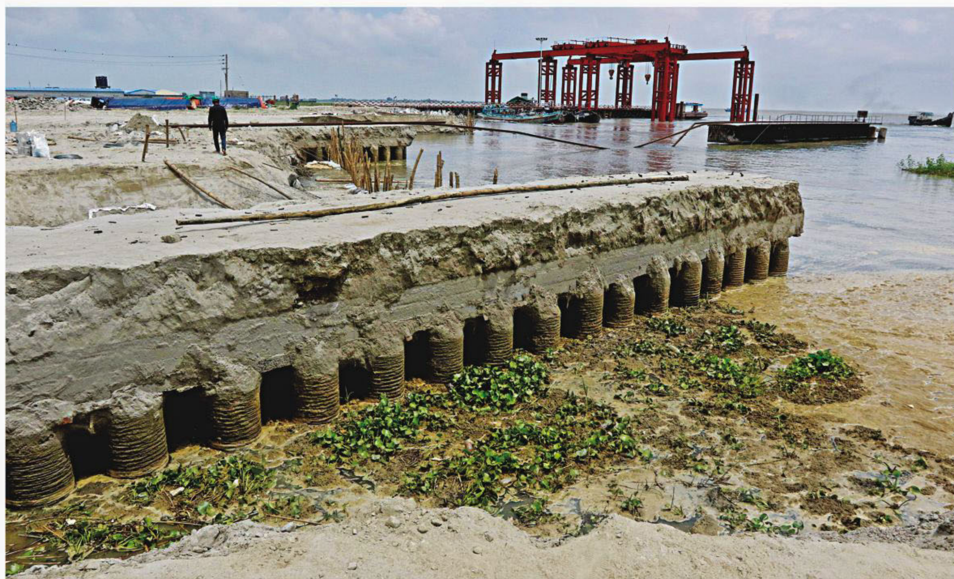
Large portions of two jetties at Padma bridge construction yard are eroded, left, and construction materials devoured, bottom right, by strong currents. Workers, top right, were seen trying to stop the erosion by putting sandbags on the banks, but to little use. The photos were taken yesterday.
