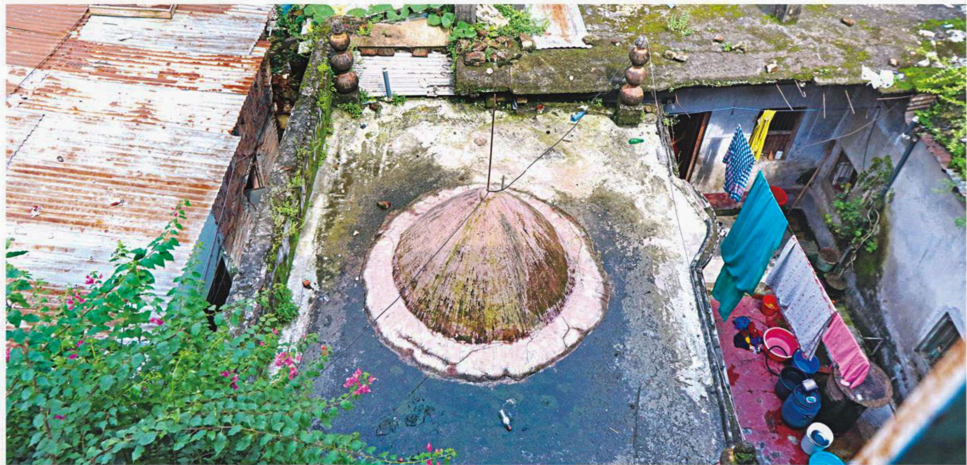
The domed roof of a shrine inside the compound of Islamia UP Government Primary School in Sutrapur. Teachers and members of the school managing committee allege that it was built with intent to grab the school land. The photo was taken yesterday.
