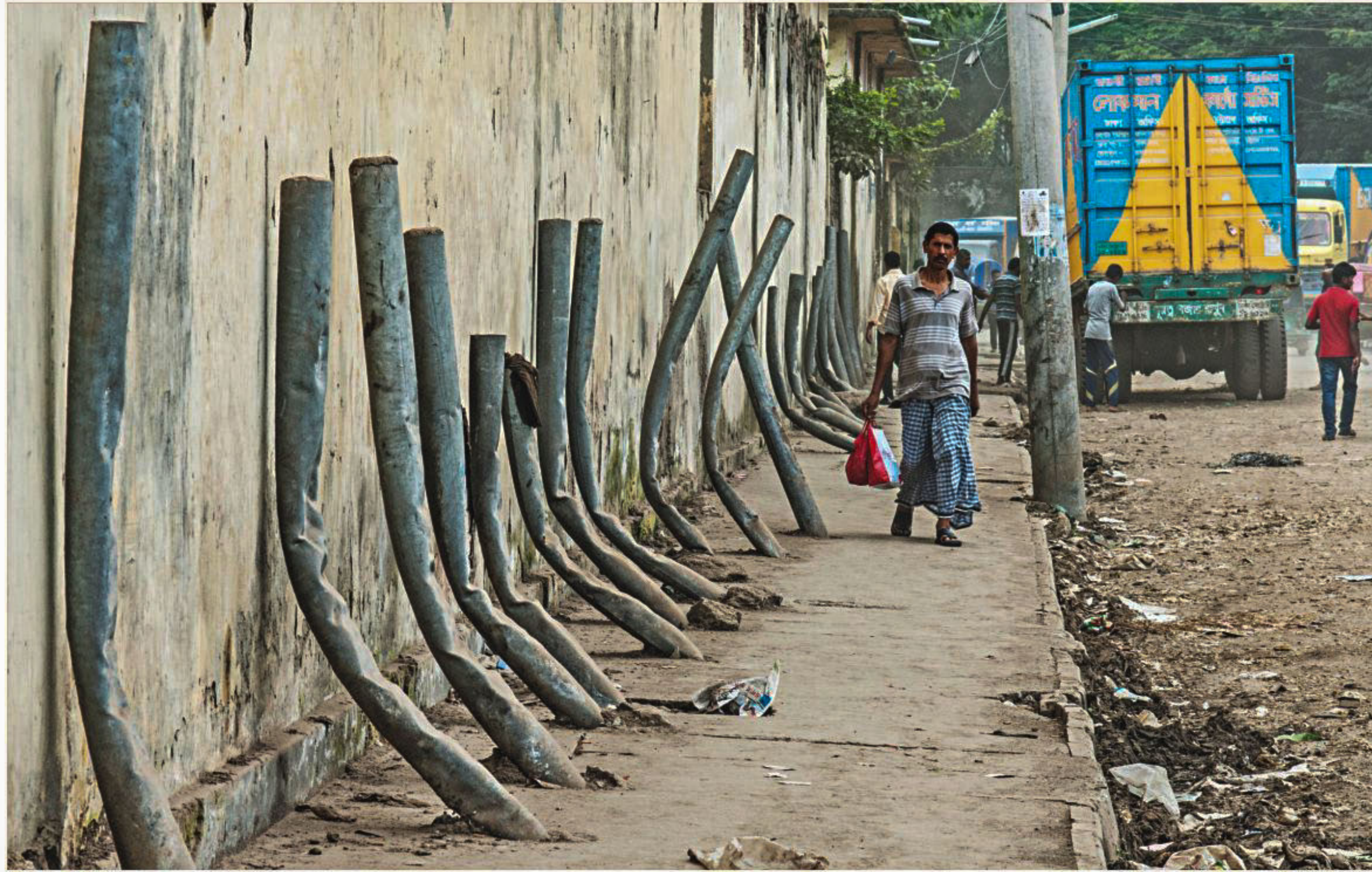
The authorities of a building in Tejgaon installed metal poles in the pavement to protect the wall from trucks that are usually parked there. The bent poles tell how overzealous the truckers are in making the pavement unusable for pedestrians.
