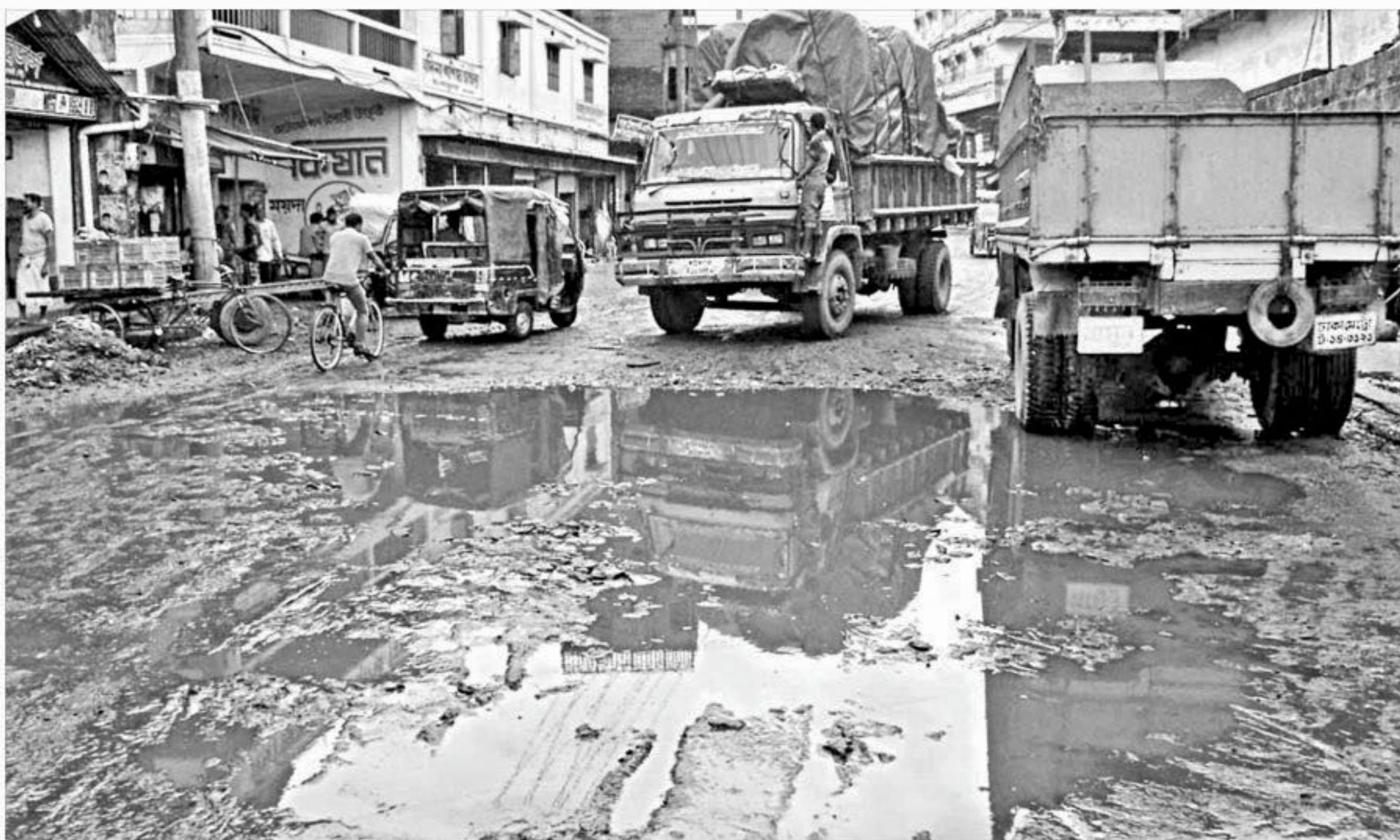
Recent rainfall in Barisal city has left most of the roads filled with craters and potholes, making it difficult for vehicles to ply, and causing sufferings to commuters. The photo was taken on Sadar Road yesterday.
