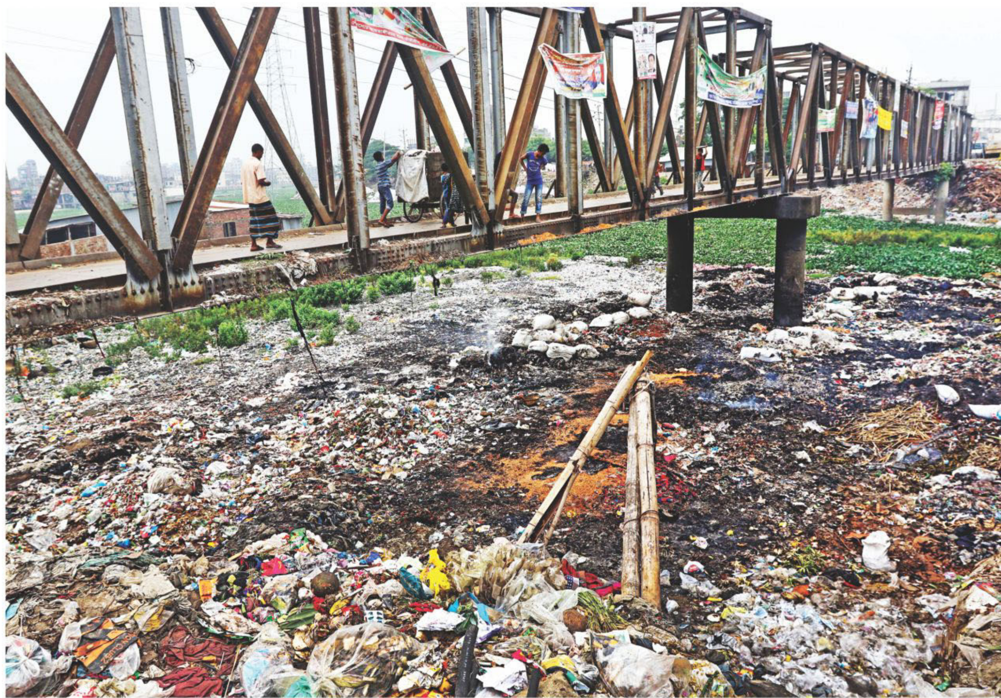
RIVER OR DUMP YARD? Waste materials dumped by locals of Kamrangirchar on the outskirts of the capital filled this channel of the Buriganga river under the Iron Bridge to such an extent that not even an inch is left for water to pass through. The photo was taken yesterday.
