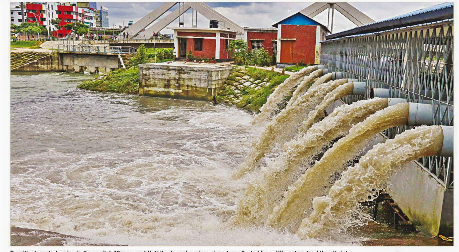
To mitigate waterlogging in the capital, 10 pumps at Hatirjheel are dumping rainwater collected from different parts of the city into a canal in Rampura that meets the Balu River. The pumps, built by Wasa and maintained by the Bangladesh Army, get water from Hatirpool, Dhanmondi, Lalmatia, Gulshan, Tejgaon and Moghbazar areas. The photo was taken yesterday.
