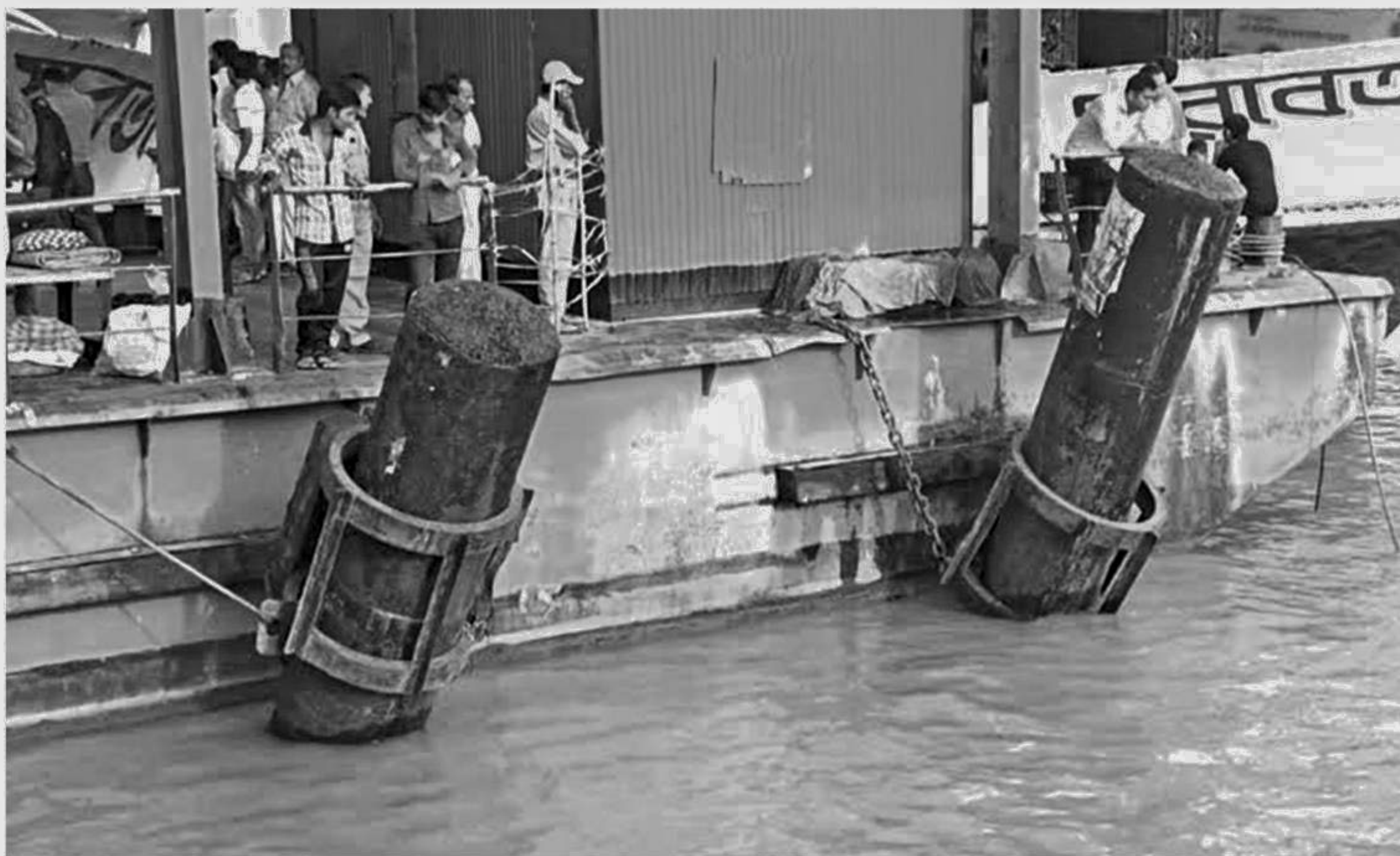
These two concrete supports of a pontoon at Barisal River Port have been dislodged after a triple-decker launch, MV Kirtankhola-2, loaded with passengers, hit those at a "high speed" during berthing on Tuesday afternoon.
