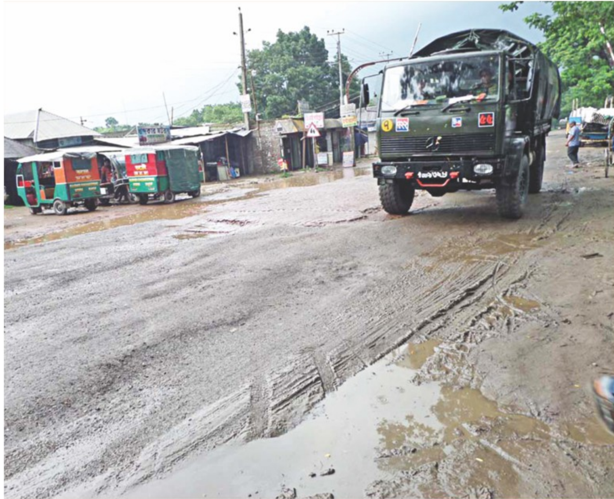
The Faridpur-Jessore highway is left in a dilapidated condition. Numerous potholes have appeared on the 43km stretch of its Faridpur-Magura part. Several points of the highway get muddy whenever it rains. The situation is likely to worsen further in the coming days as hundreds of vehicles, taking millions of Eid holidaymakers home, will hit the highway. The pictures were taken six days ago.
