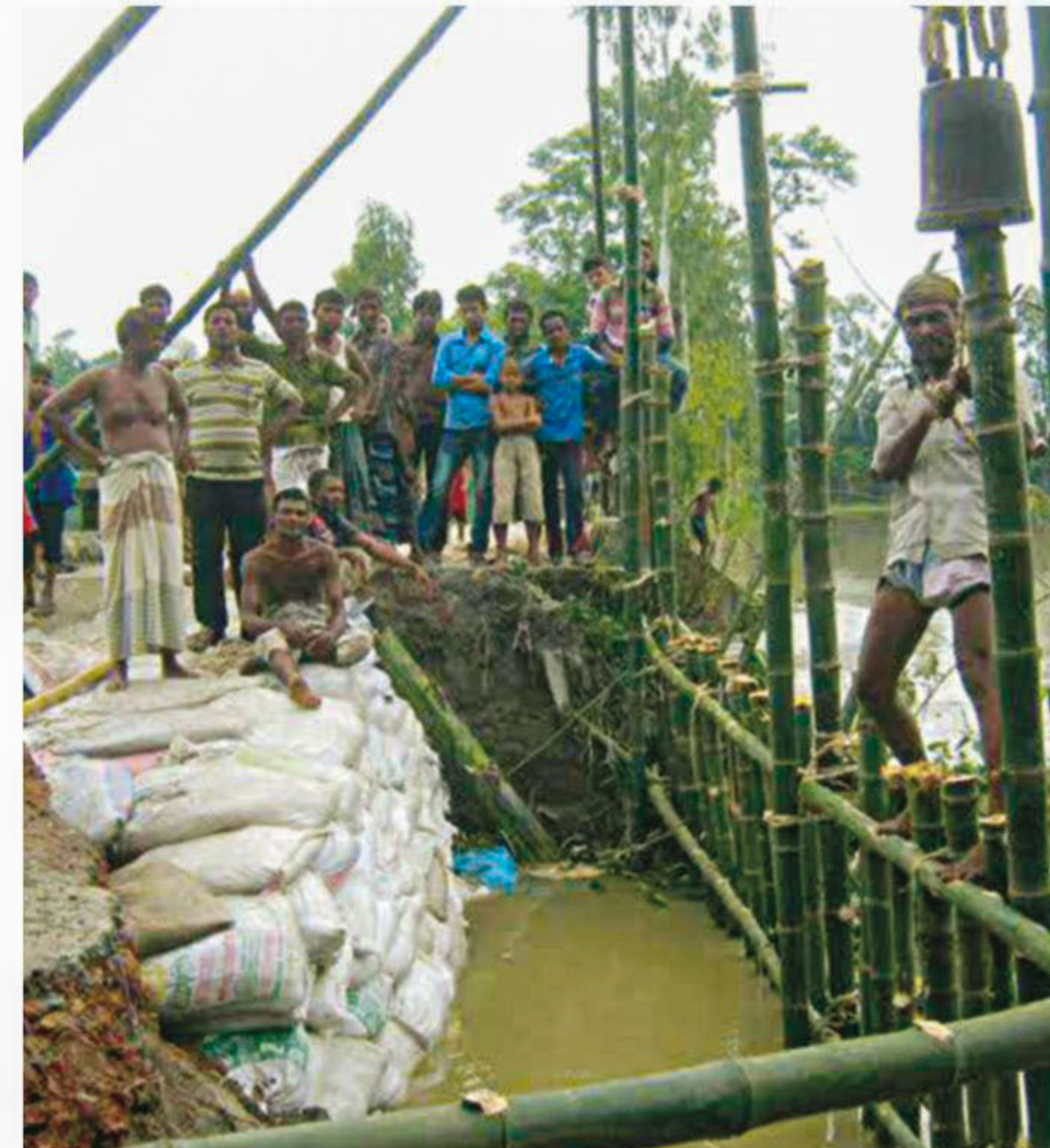
Villagers build an embankment with bamboo piling to save Barakata bypass from erosion by the Teesta River in Hatibandha upazila of Lalmonirhat district. The photo was taken on Monday.
