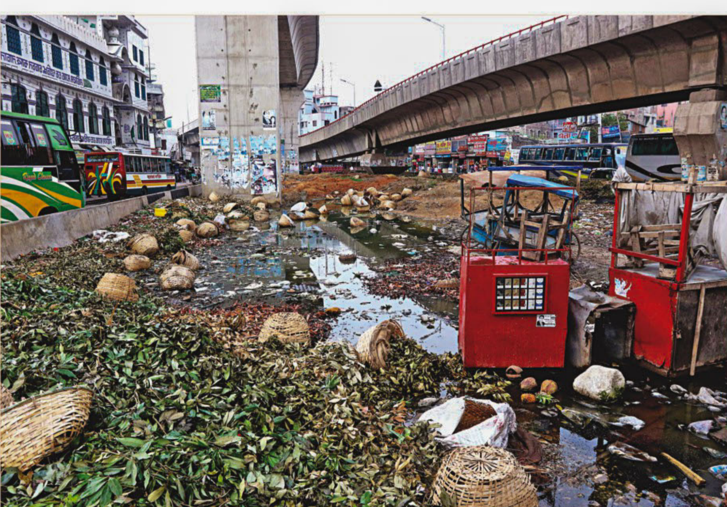
Garbage floating on rainwater gives a patch under Mayor Mohammad Hanif Flyover at the capital's Sayedabad a resemblance to a badly managed dumping ground, causing sufferings to commuters. However, the authorities are nonchalant. The photo was taken last week. PHOTO: ANISUR RAHMAN
