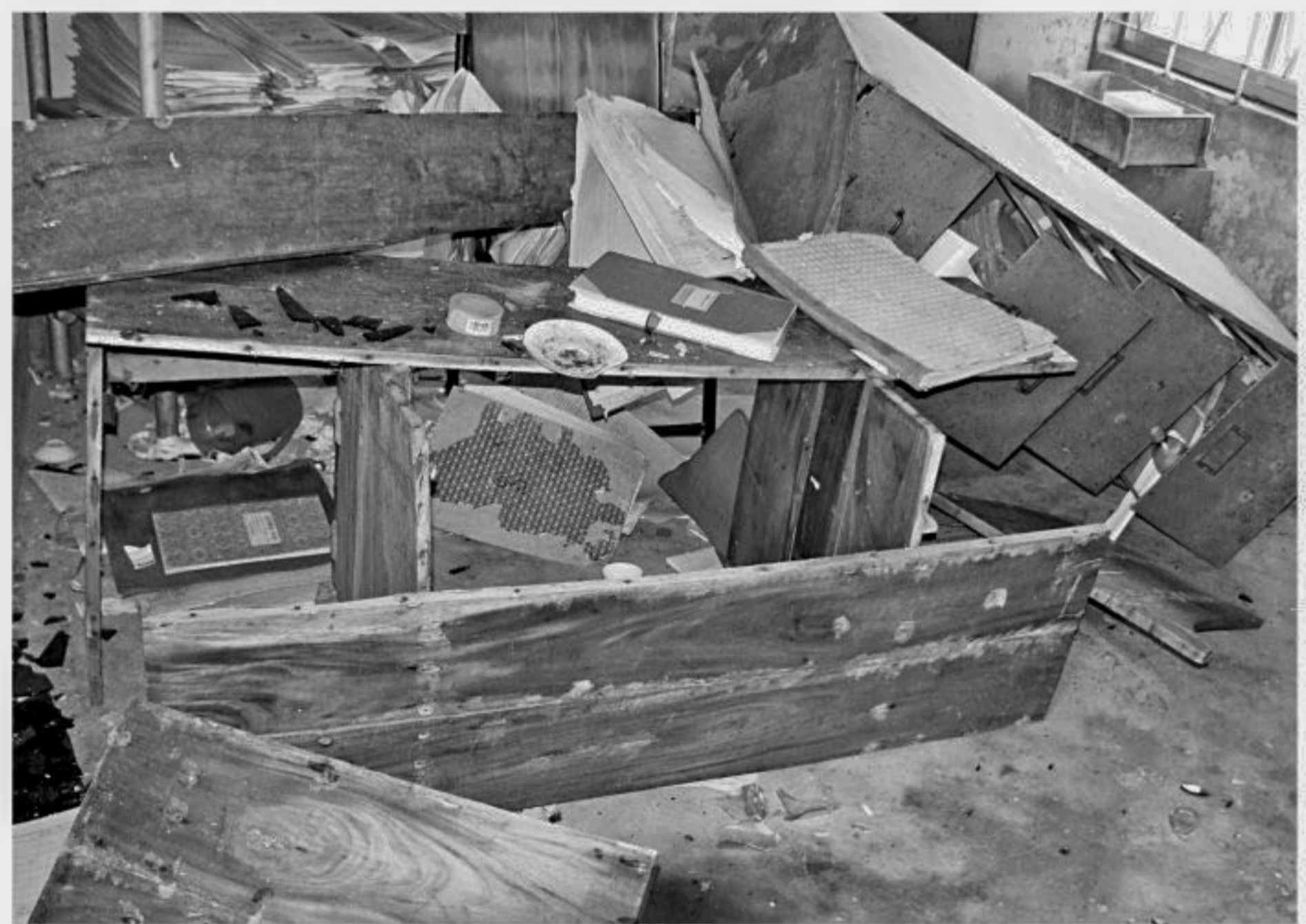
PHOTO: STAR Aggrieved locals vandalise the West Zone Power Distribution Company office in Charfashion municipality yesterday protesting frequent power outage in the upazila under Bhola district.
