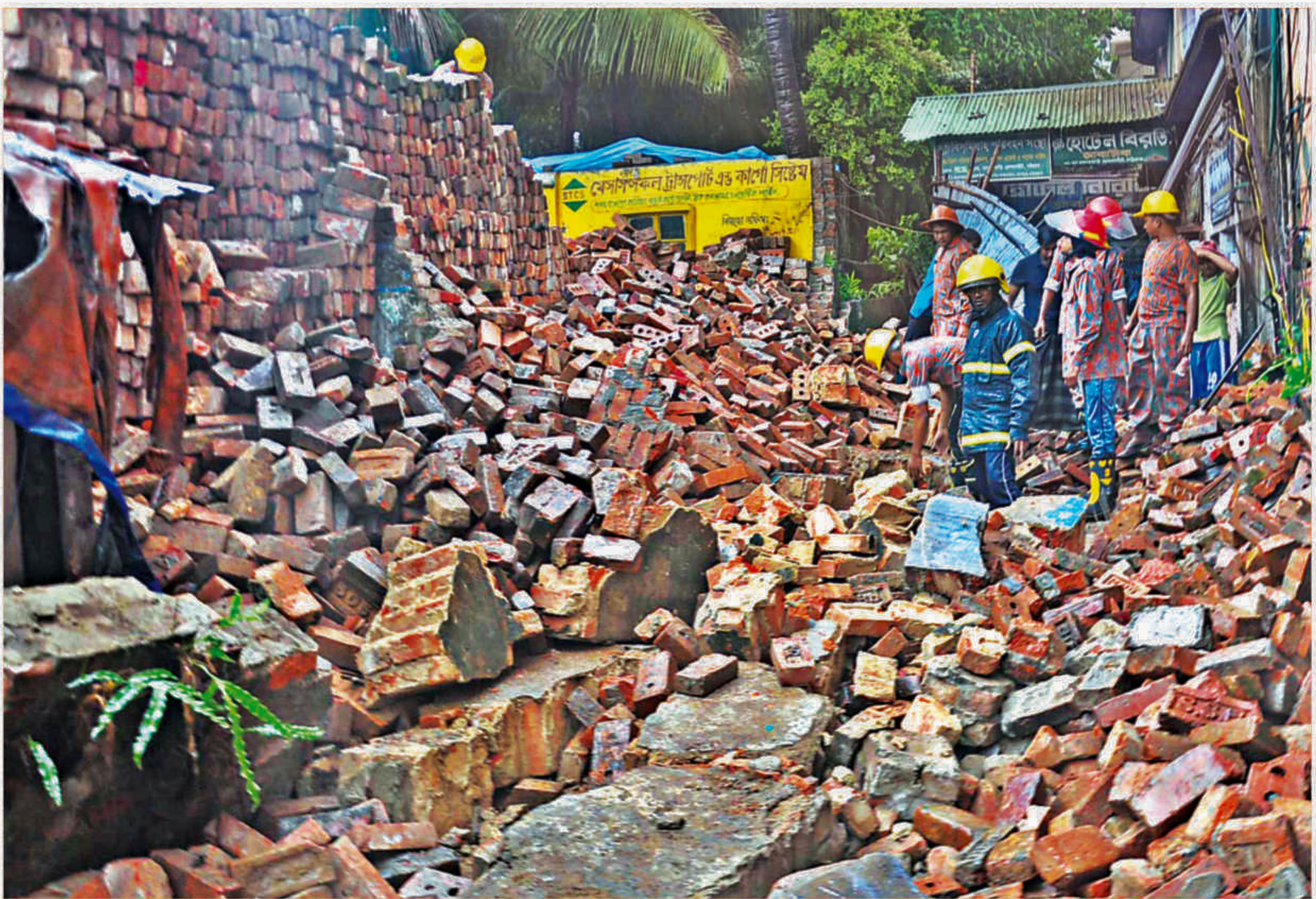
Rescuers work through the rubble at a wall collapse site at East Madarbari of Chittagong city yesterday.
