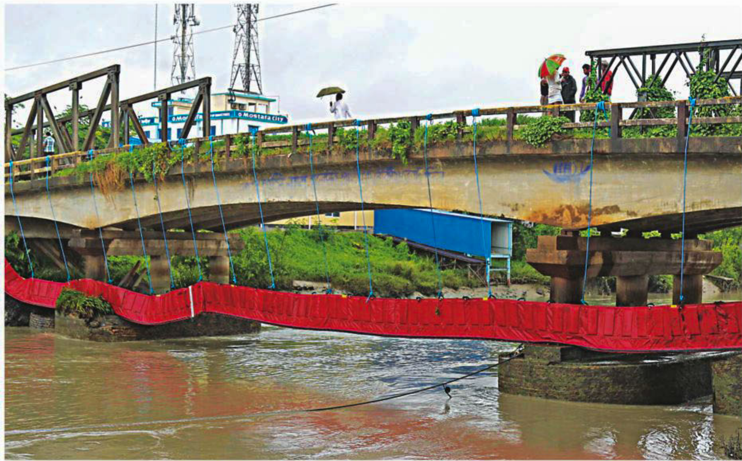
An oil-boom, used for containing oil spill, hangs from a bridge in Shakpura area of Chittagong. The barrier was placed two feet above the water level two days after three oil wagons of a train fell into a canal at Khatibchar. The oil-boom was installed to prevent oil from flowing into the Karnaphuli river, but it was of no use as oil had already spread to the river.
