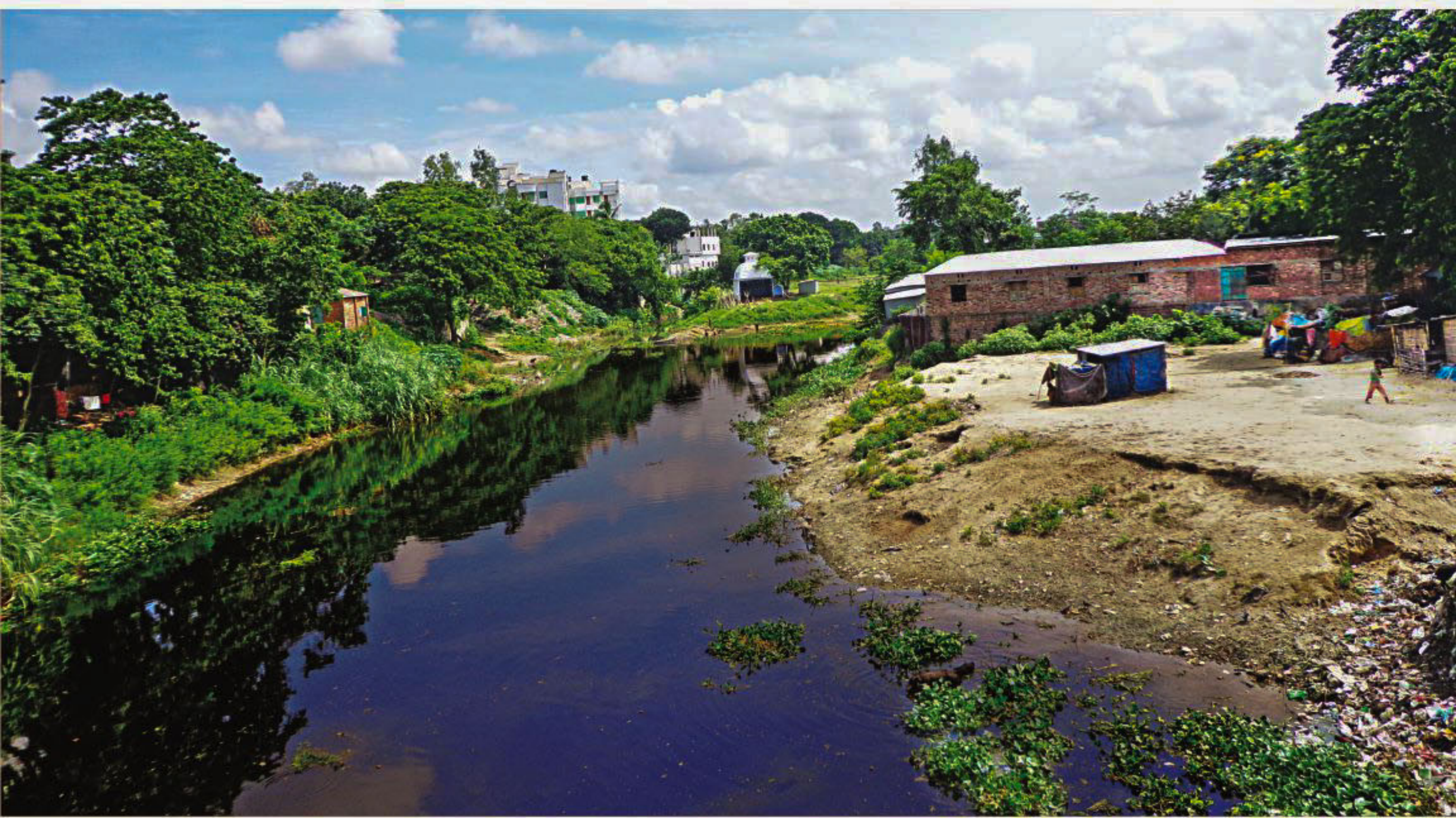
Encroachment and pollution are slowly destroying the Karatoa river, by narrowing it from both banks, blocking its natural flow, and poisoning the water. Against the backdrop, the High Court yesterday ordered the authorities to immediately stop dumping of waste into the river and to take necessary steps to protect it from encroachment. The photo was taken near Bogra town recently.
